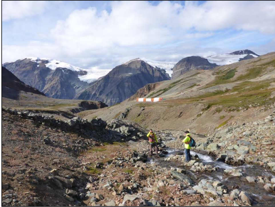
Image 5: View west to tailings dam from Goldslide Creek.
