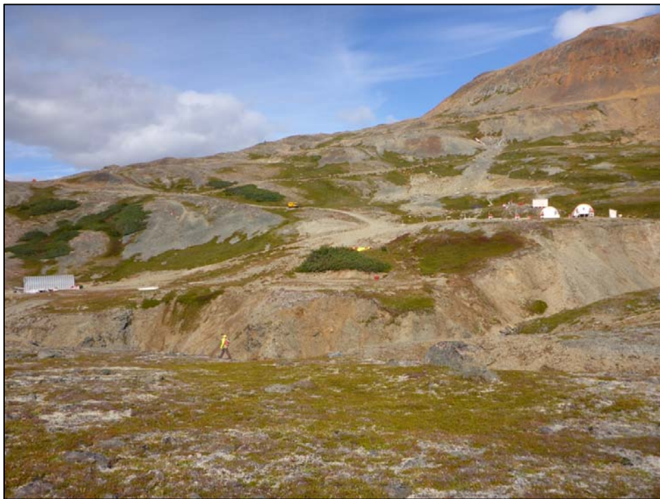
Image 6: View north from south of Goldslide Creek at proposed tailings dam showing general terrain; proposed mill site at upper left.
