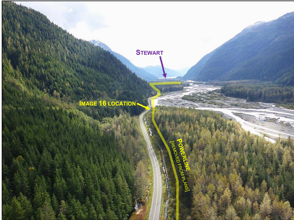
Image 17: Aerial view south over Highway 37A, the Bear River, and previously proposed powerline (approximate centreline).
