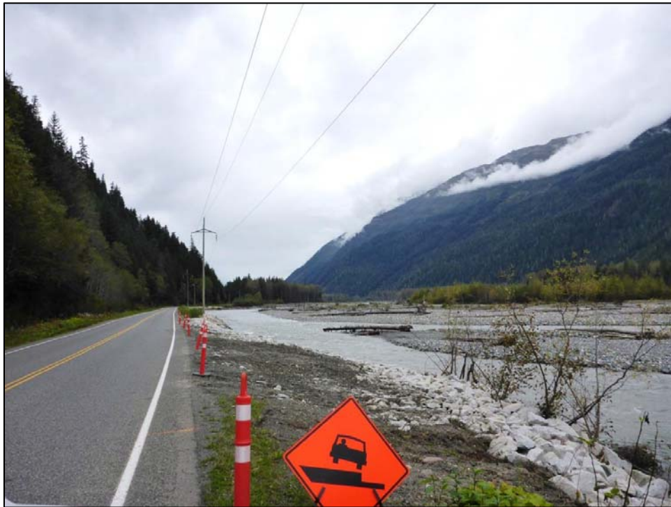
Image 16: View south to Bear River and Highway 37A washout.
