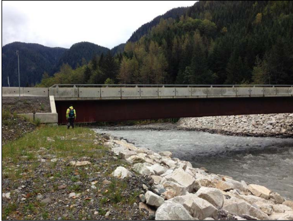
Image 15: View east (upstream) to Highway 37A at Bitter Creek Bridge.
