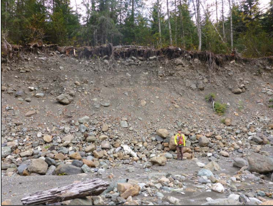
Image 11: View of east bank of Bitter Creek, south of Roosevelt Creek, showing significant natural erosion of remnant terrace.
