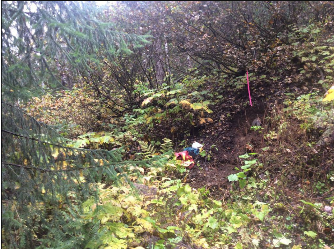
Photo 4c – Steep slope above existing road alignment 1km east of Roosevelt Creek.
