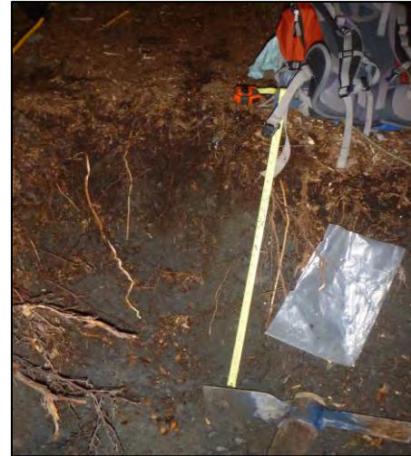
PHOTO 22 BH16-004 Hand Dug Test Pit
