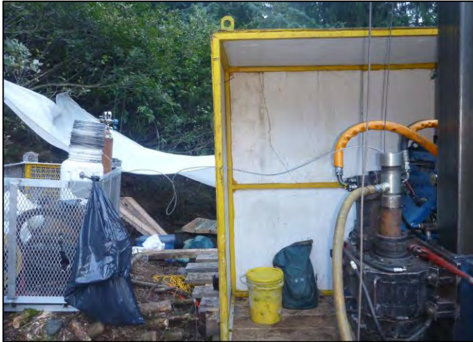
PHOTO 17 BH16-004 Nitrogen Packer Gas Tank Setup
