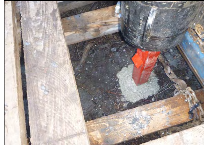
PHOTO 65 MW16-003 Completed Standpipe Installation
