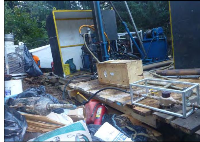
PHOTO 18 BH16-004 Nitrogen Packer Assembly
