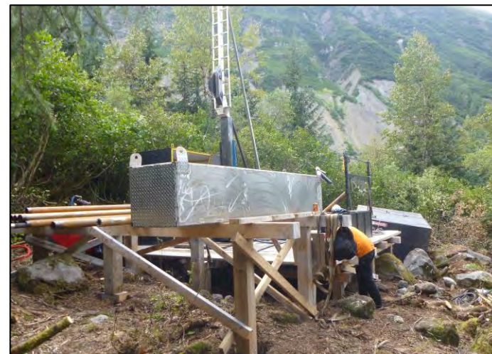
PHOTO 52 MW16-001 Looking West
