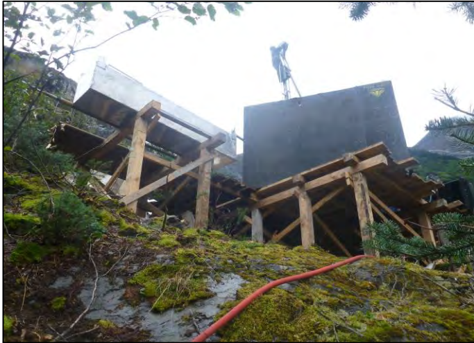
PHOTO 37 BH16-008 Looking North
