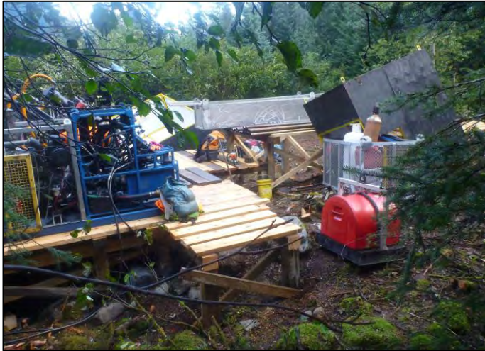
PHOTO 9 BH16-003 Looking North
