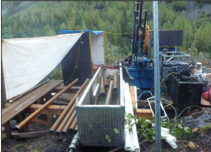
PHOTO 41 BH16-009 Looking North
