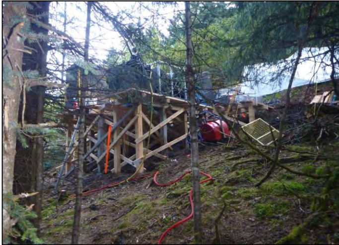
PHOTO 13 BH16-004 Looking North
