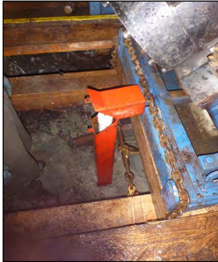
PHOTO 57 MW16-002 Completed Standpipe Installation
