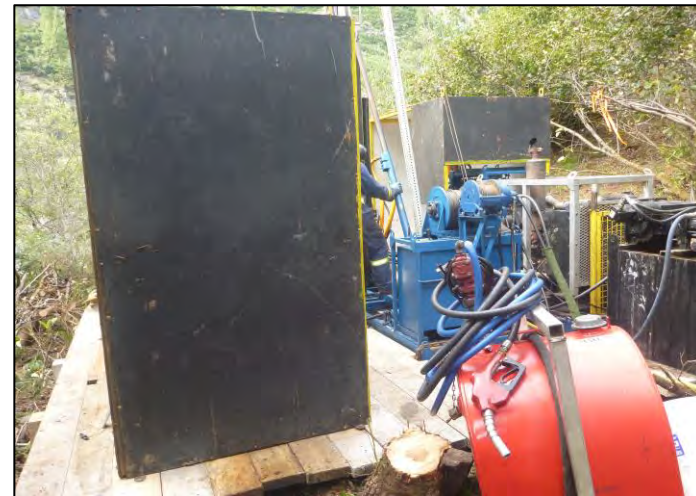
PHOTO 63 MW16-003 Looking West
