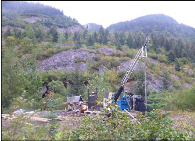
PHOTO 5 BH16-002 Looking North
