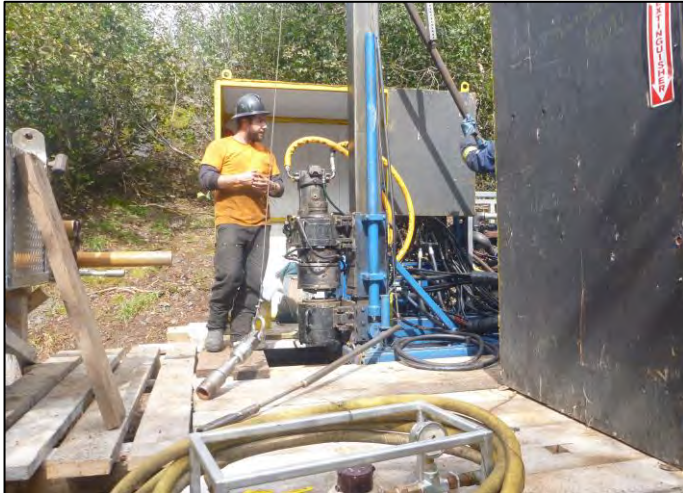
PHOTO 60 MW16-003 Looking North
