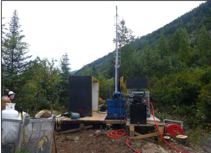
PHOTO 1 BH16-001 Looking North
