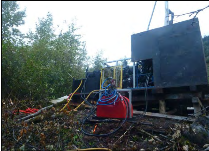
PHOTO 31 BH16-007 Looking North
