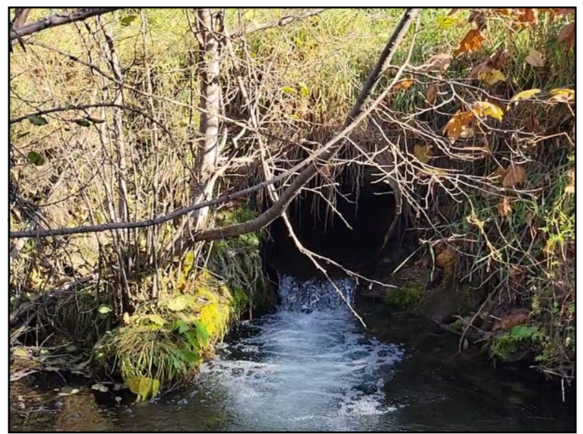
Photo 2 Hanging culvert outlet at Grace Creek Crossing 1.
