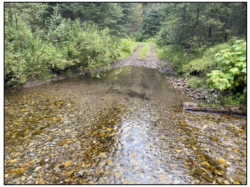
Photo 1 Left bank of truck ford showing erosion and sedimentation.
