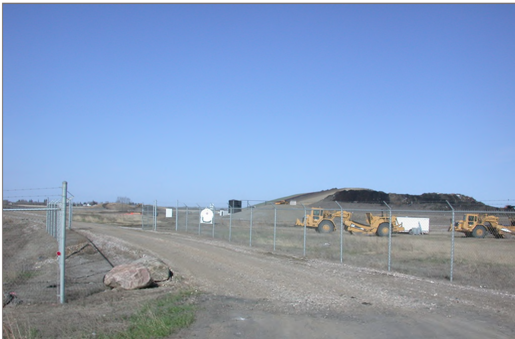
Photo 2: View northwest towards the existing landfill cells from Secondary Highway 854.
