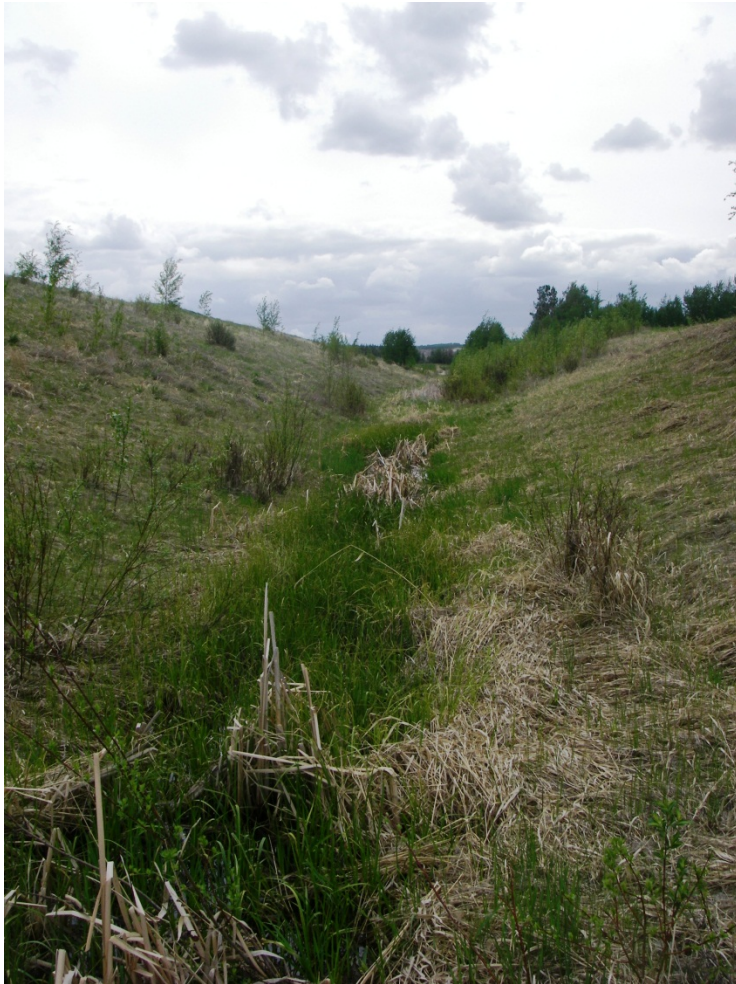
Photo 3: South portion of an interceptor ditch that runs north-south through the Project site, facing south. Vegetation is mostly dominated by grasses and shrubs with occasional patches of regenerating aspen and balsam poplar.
