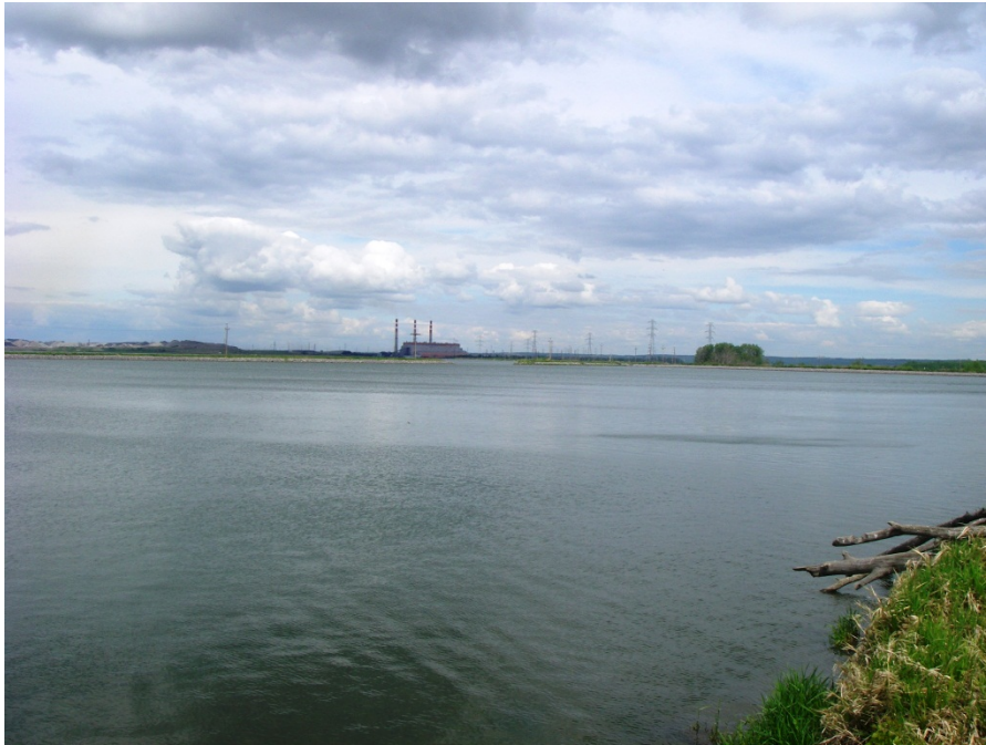
Photo 5: Sundance Industrial Cooling Pond facing northwest towards the Sundance Thermal Electric Power Plant and existing transmission facilities.
