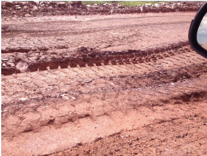
Figure 4-2: Photos of Recent Thawing of Frozen Ground – Active Layer or Permafrost Degradation
