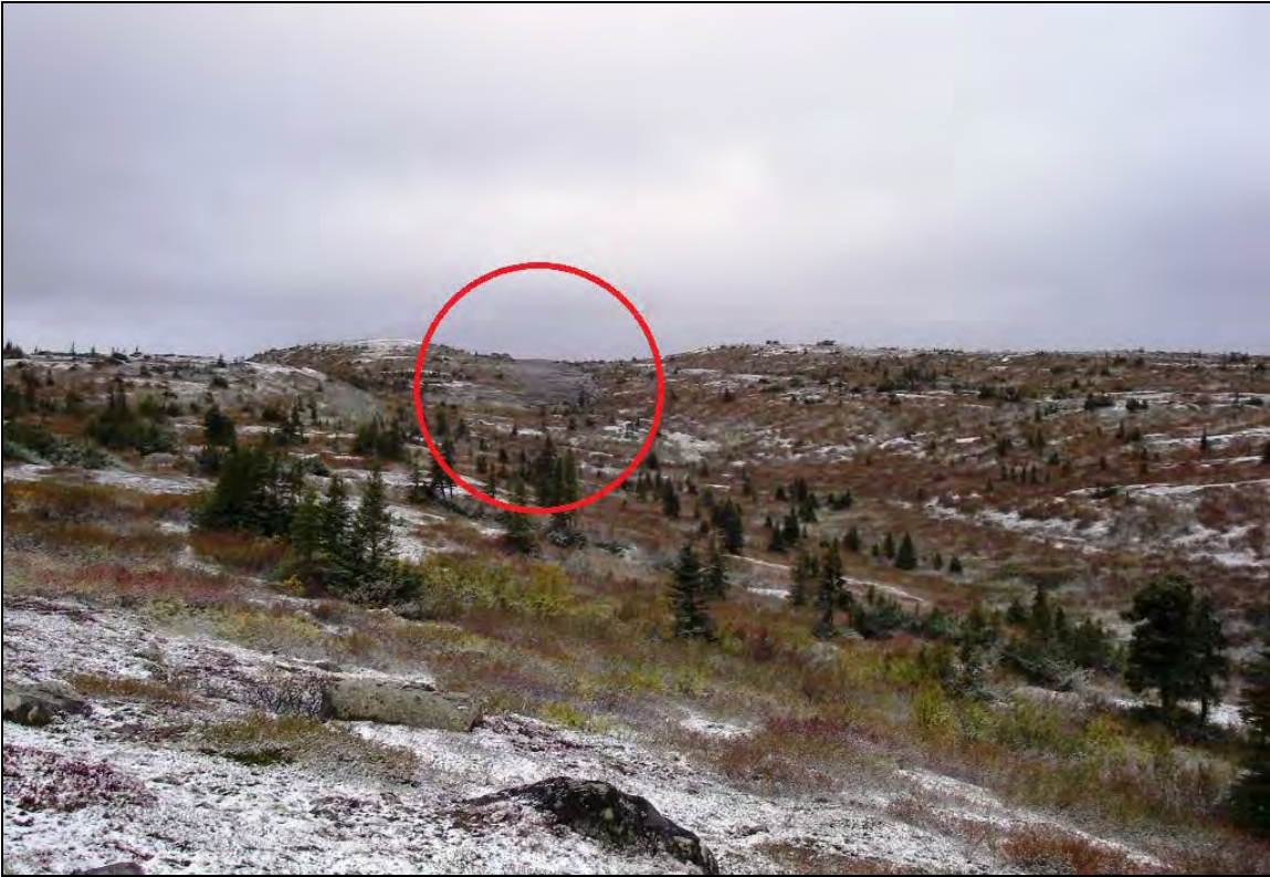
Goodwood-Timmins haul road construction, viewed from NW end of SA3.
