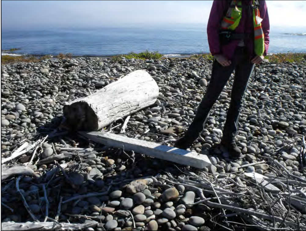
Plate 16: A displaced Crown land marker on the cobble beach, looking east.
