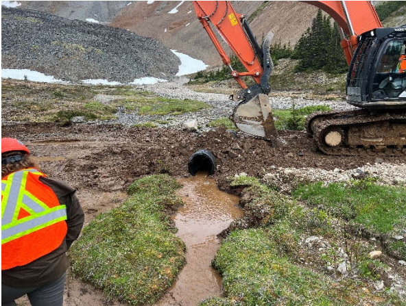
Plate 009: Culvert 1 at site KN002.
