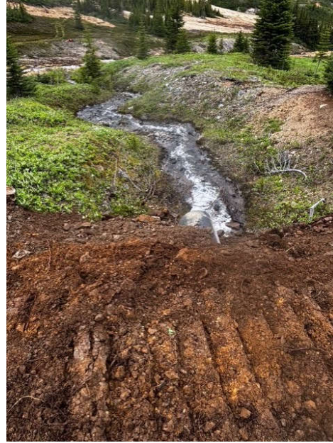
Plate 020: Final installation of temporary crossing at KN003.
