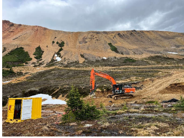
Plate 002: Site prep for structure installation and site KN001.
