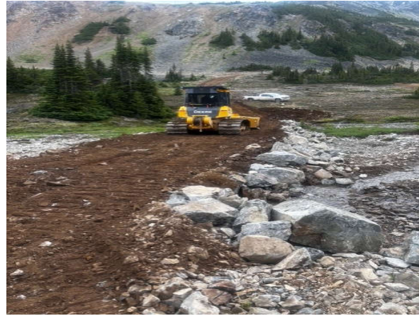
Plate 010: Completed works at crossing site KN002.
