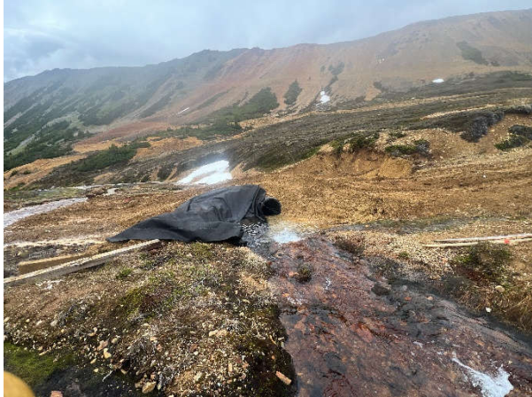
Plate 007: Geofabric installation at inflow of 900mm culvert at site KN001.
