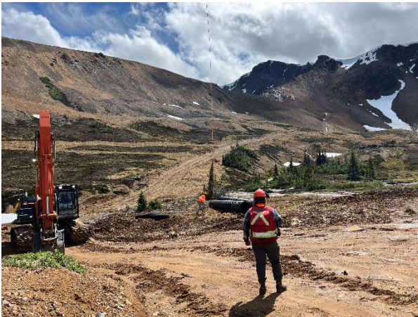
Plate 003: Site prep for structure installation at crossing KN001.
