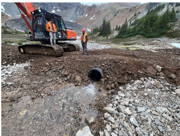
Plate 013: Culvert 2 outflow at crossing site KN002 with riprap armouring placement.
