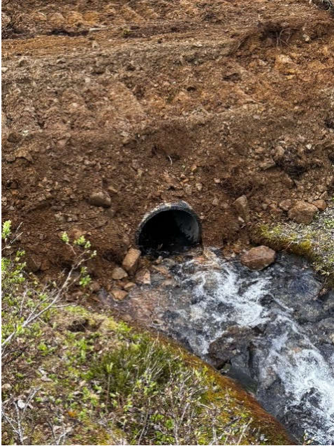
Plate 019: Final installation of temporary crossing at KN003.
