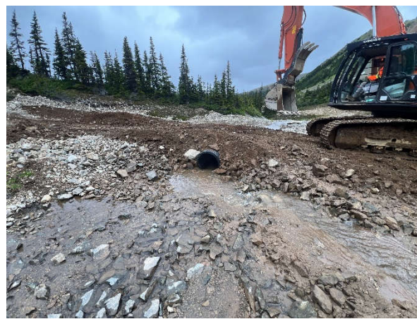
Plate 014: Culvert 2 inflow at crossing site KN002 with riprap armouring placement.
