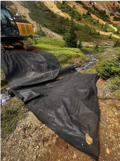
Plate 017: Installation of geofabric at temporary crossing KN003.
