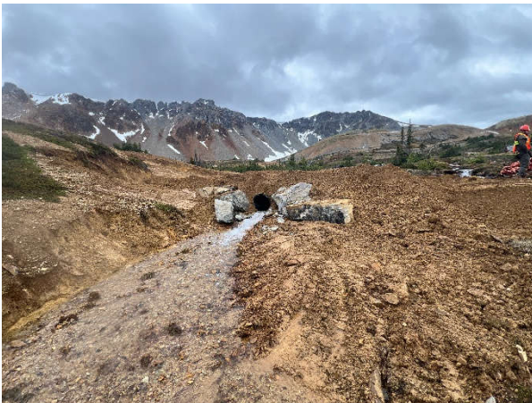
Plate 005: Riprap armouring at outflow of crossing at KN001.
