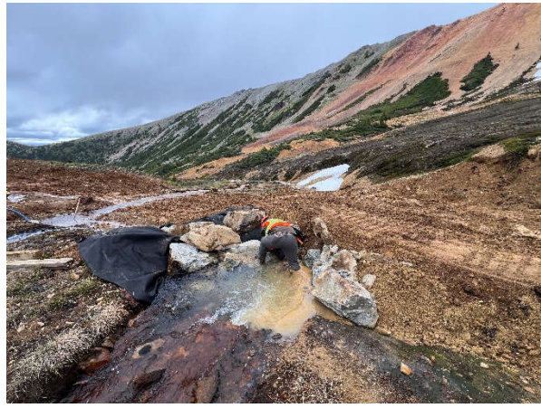
Plate 004: Geofabric and riprap armouring at inflow of crossing site KN001.
