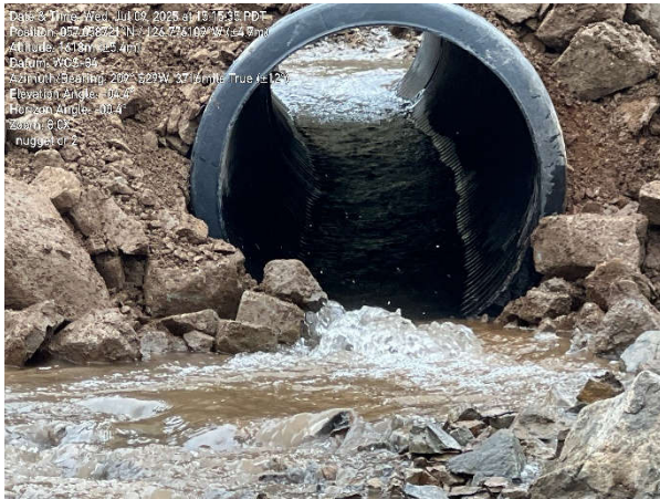
Plate 011: Culvert 2 inflow at crossing site KN002 with riprap armouring placement.
