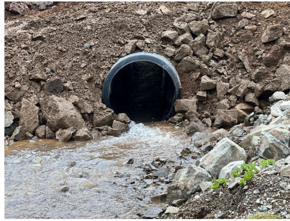
Plate 012: Culvert 2 inflow at crossing site KN002 with riprap armouring placement.
