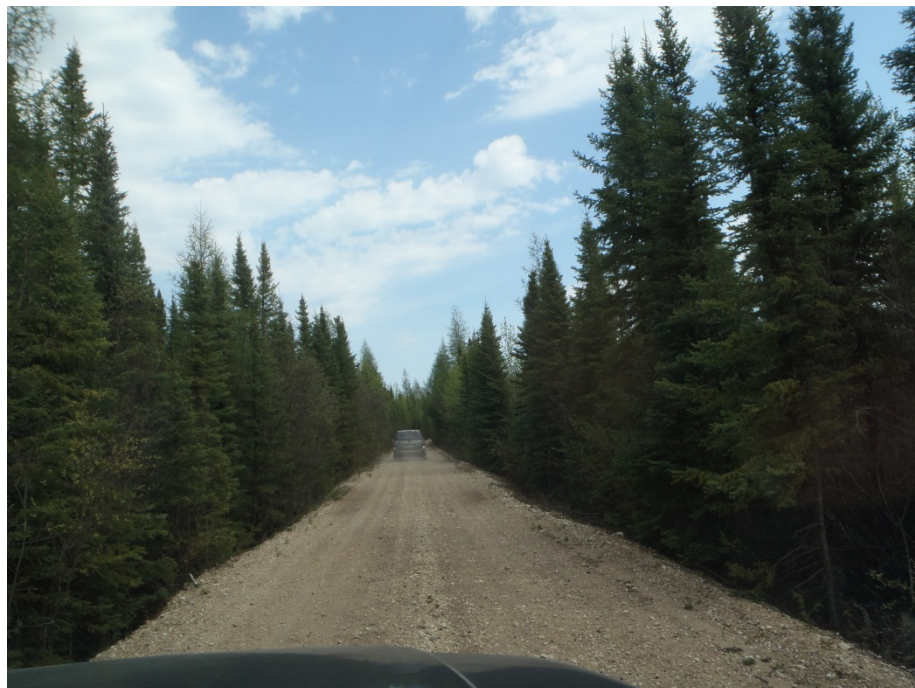
Photo 4: Corridor of the Pipeline System (along the former rail bed).
