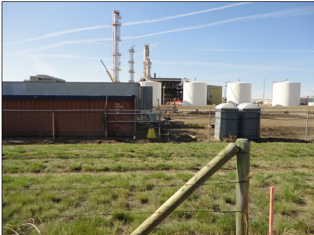
Figure 8 - South-Central Location Viewing South (existing Methanex infrastructure in background)
