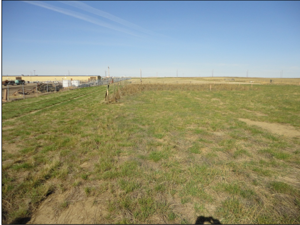
Figure 7 - South-Central Location Viewing West (existing Methanex infrastructure in background)
