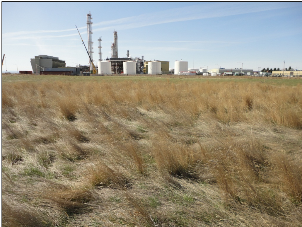
Figure 16 - Central Location Viewing South (existing Methanex infrastructure in background)
