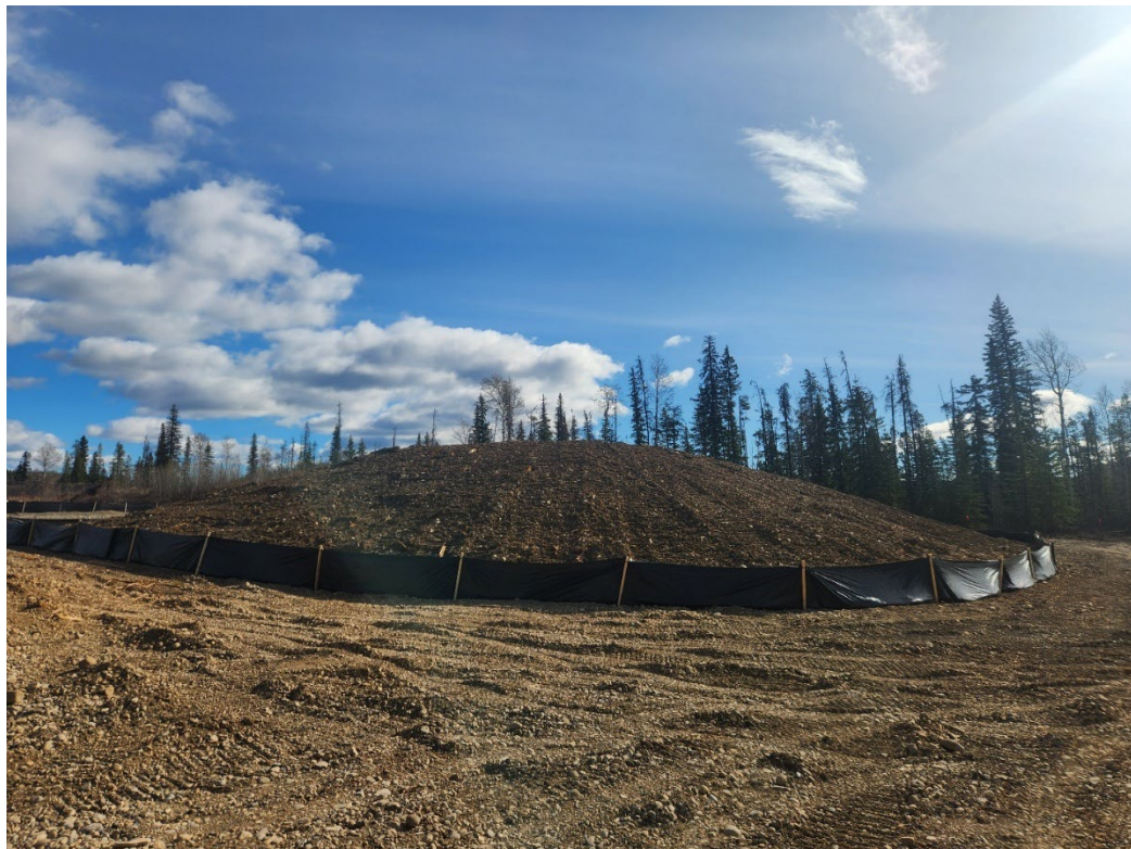
Appendix Photo A-6. Topsoil stockpile at the decline site after tree clearing activities at its long term location (April 23, 2025).
