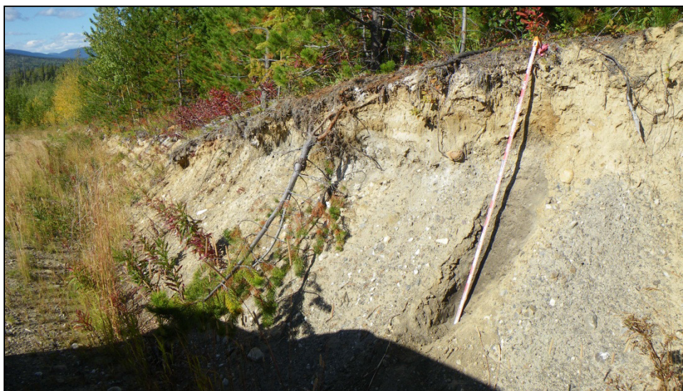
Plate 4.3-15. The soil profiles of SMU-GF2 typically feature a clear boundary between the coarser surficial horizons and the finer, more compacted, deeper morainal horizons.
