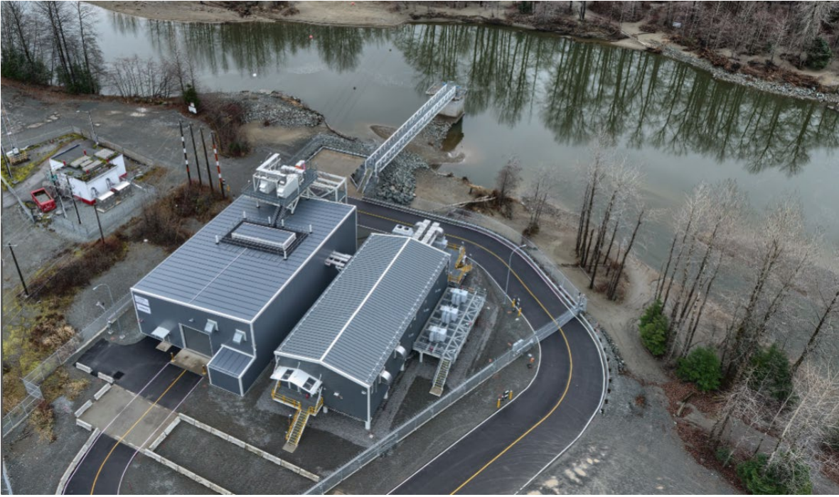
PHOTO 5: COMPLETED CONSTRUCTION OF THE RIVER WATER INTAKE (NOV 2024)
