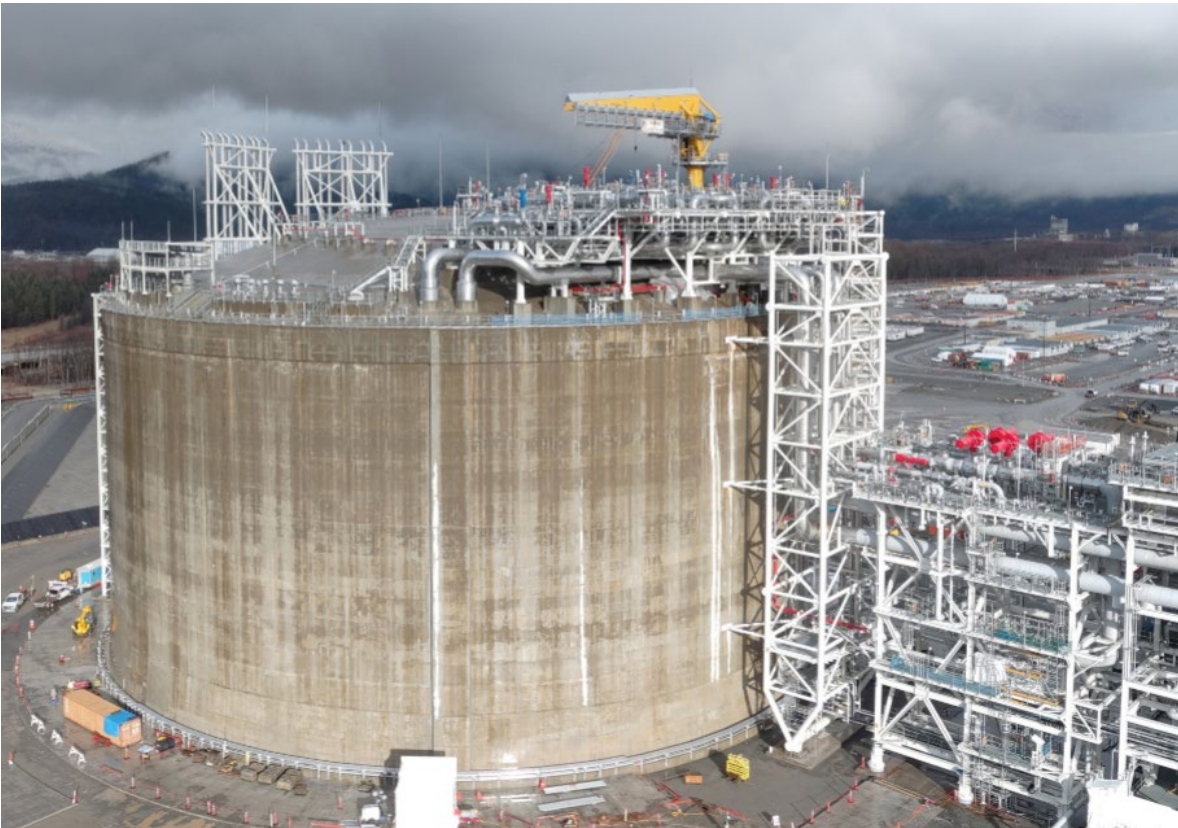
PHOTO 6: LNG TANK CONSTRUCTION COMPLETE, PREPARED FOR COOLDOWN (MARCH 2025)
