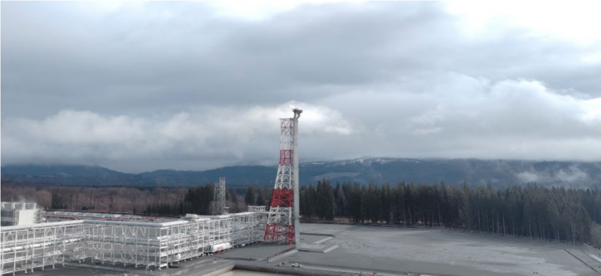
PHOTO 7: ACTIVE FLARE STACKS (MARCH 2025)
