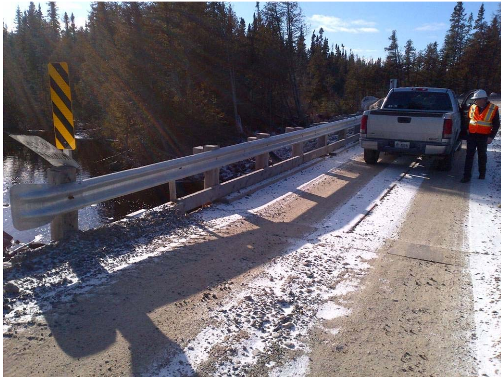
Photograph 1: Three Duck Lakes Bridge
