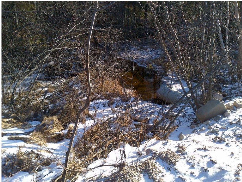
Photograph 17: Clam Lake Outlet Looking Downstream
