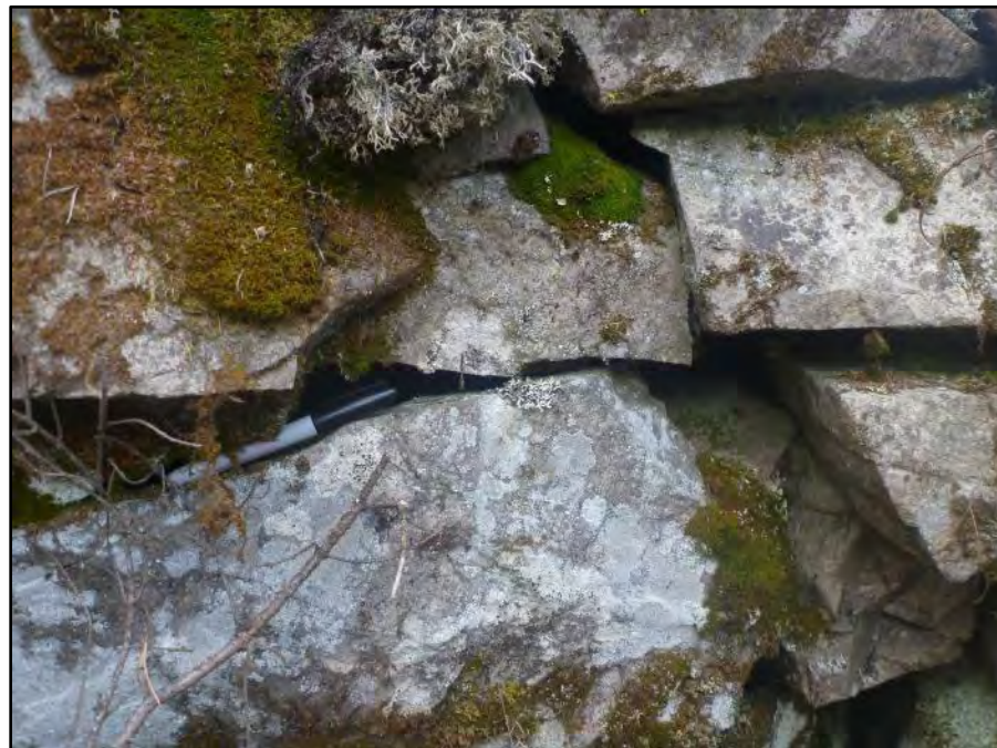
Photo 14: Crevice observed at 117lo
