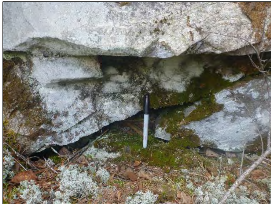
Photo 13: Crevice observed at 117lo
