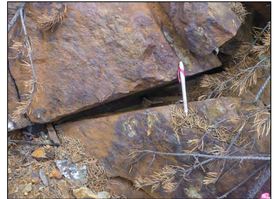
Photo 17: Crevice observed at 100med
