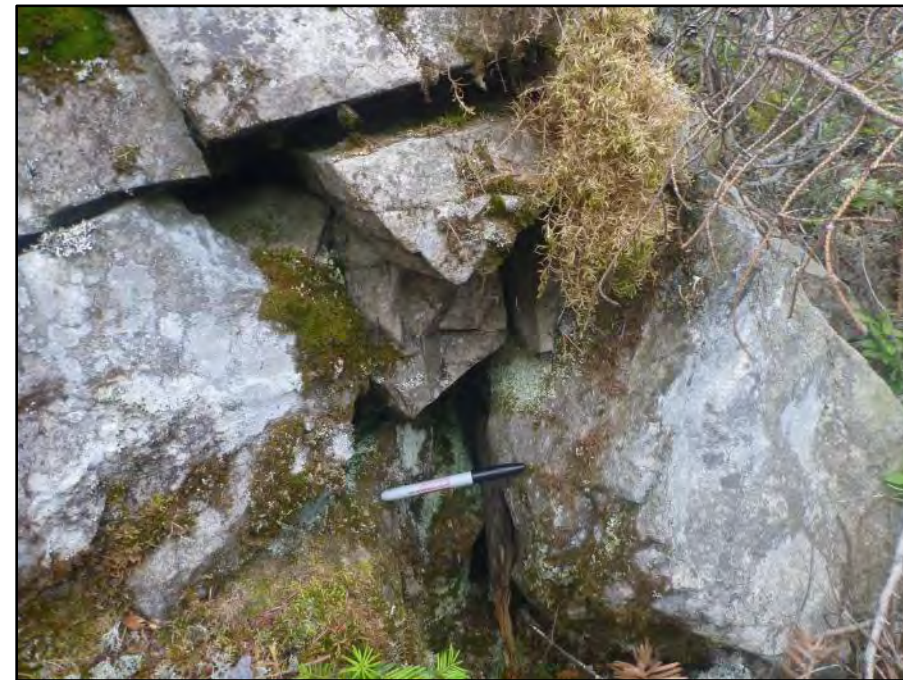
Photo 15: Crevice observed at 117lo
