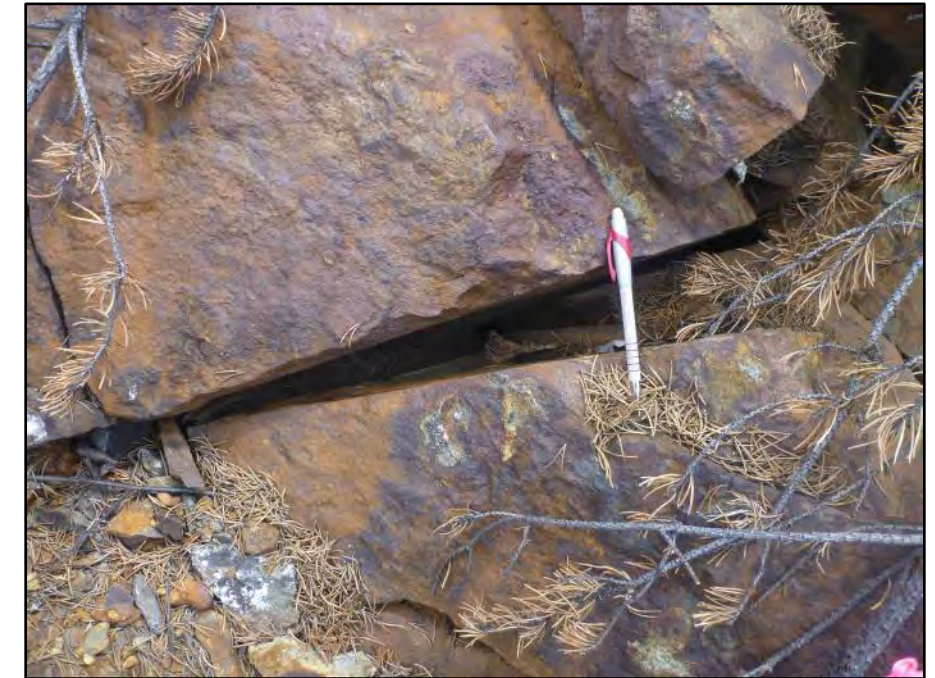
Photo 17: Crevice observed at 100med
