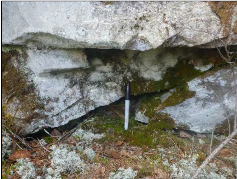
Photo 13: Crevice observed at 117lo
