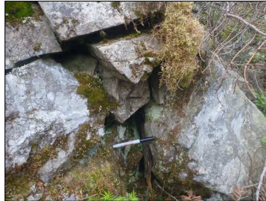
Photo 15: Crevice observed at 117lo
