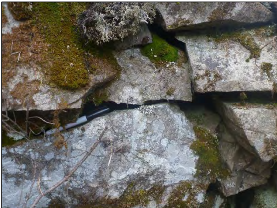
Photo 14: Crevice observed at 117lo
