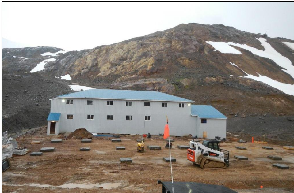
Plate 30.3-4. View of Brucejack Mine Site area activity showing exposed surface materials.
