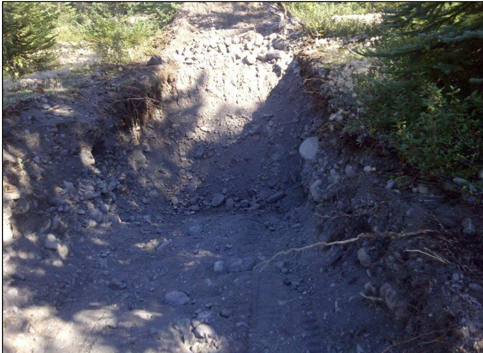
Plate 30.4-6. Gravelly soils and subsoils occurring in the Bowser Aerodrome site.
