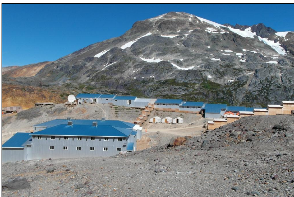
Plate 30.5-2. Bunkhouse and kitchen (large buildings in foreground) to be retained for the permanent camp.
