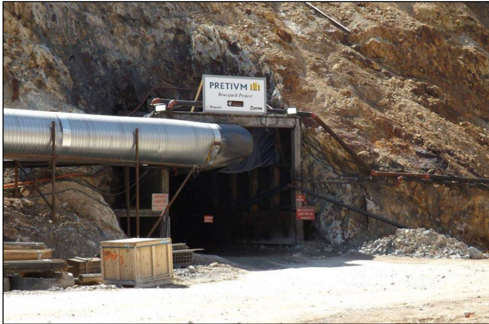
Plate 30.5-1. West Zone Portal developed by Newhawk Gold Mines and used by Pretivm for underground exploration.
