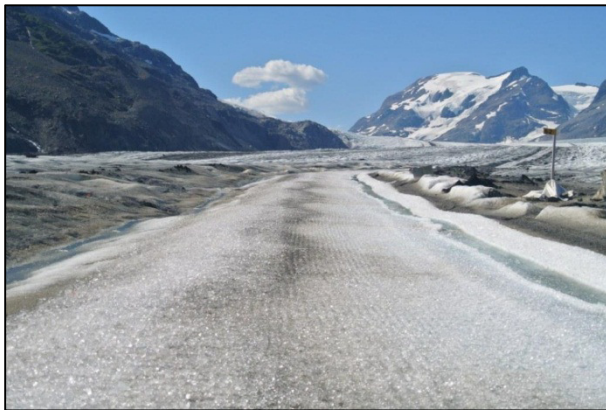
Plate 1-3. Access Road on Knipple Glacier at 62 km Section. View is towards the top of the glacier. Photo taken July 2013.
