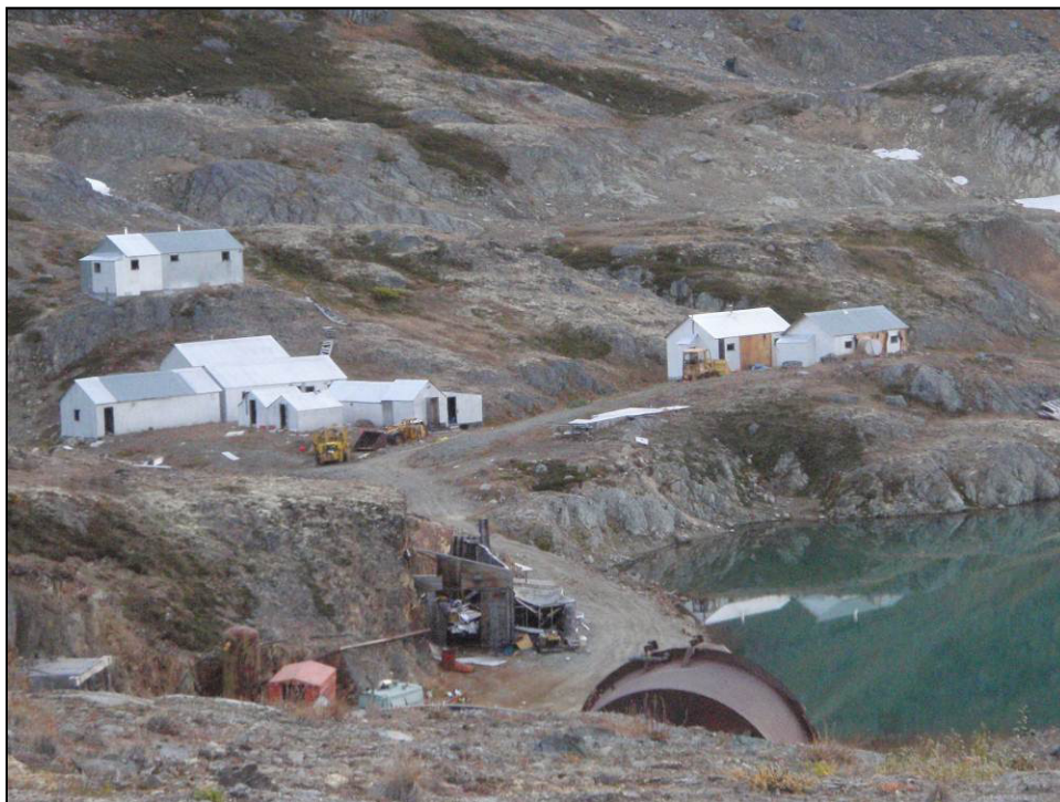
Plate 7.4-9. The abandoned Catear Resources Mine, northwest of Brucejack Lake (H-8).
