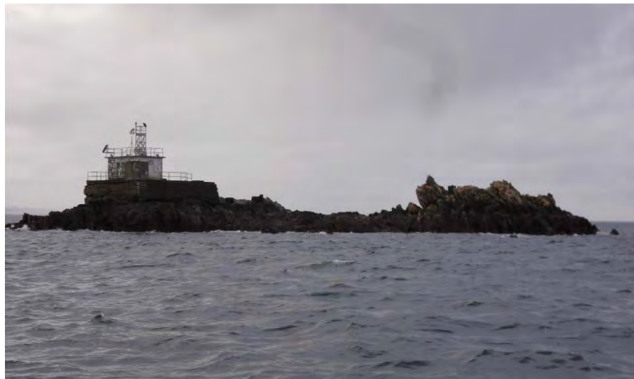
Figure G-1: Holland Rock Station (looking southwest Jan. 20, 2015)
