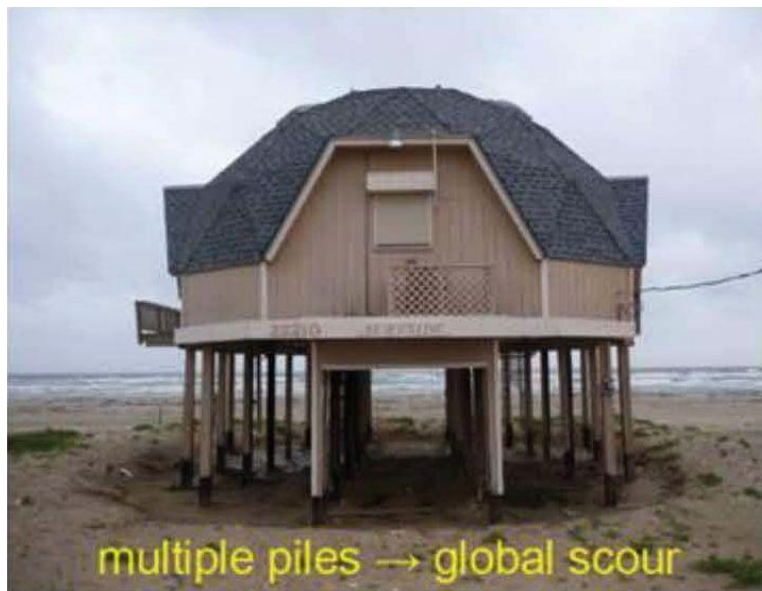
Figure 6-1: Global Scour Due to Multiple Piles [13]
