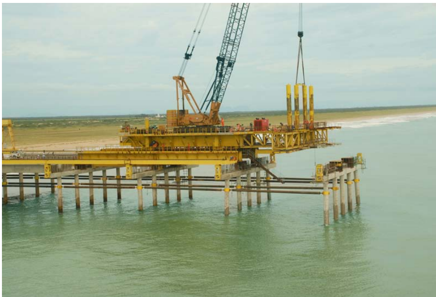
Figure 3-2: Cantilever Construction with Cantitraveler Platform
