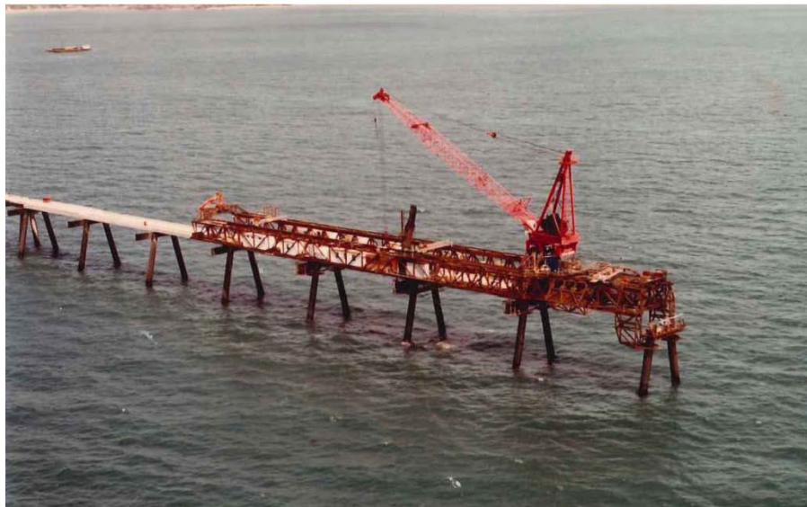
Figure 3-3: Cantilever Construction with Cantilevered Bridge
