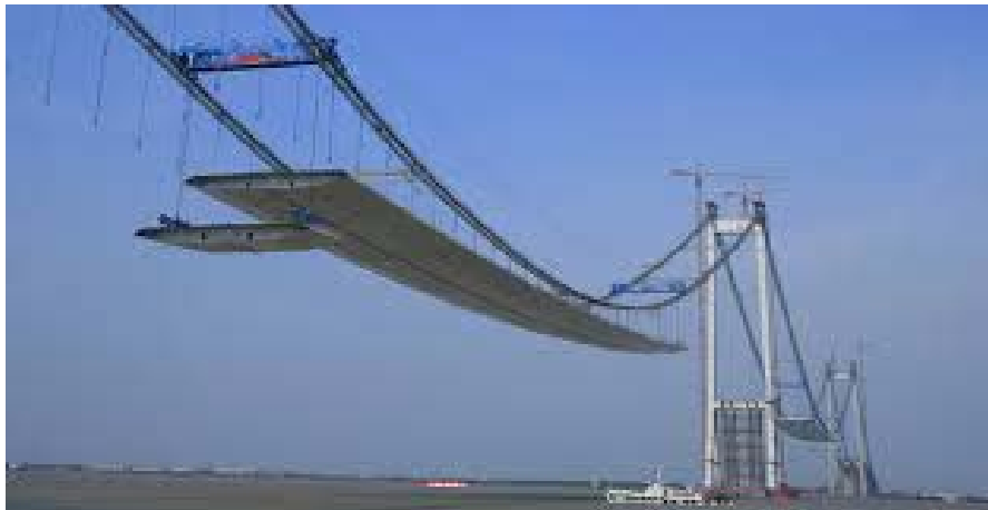
Figure 2-10: Deck Segment Installation
