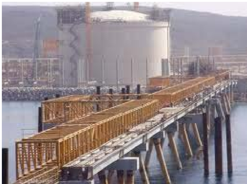
Figure 3-1: Typical LNG Trestle Structure under Construction
