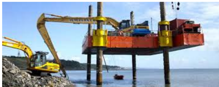
Figure 6-1: Typical Jack-up Barge
