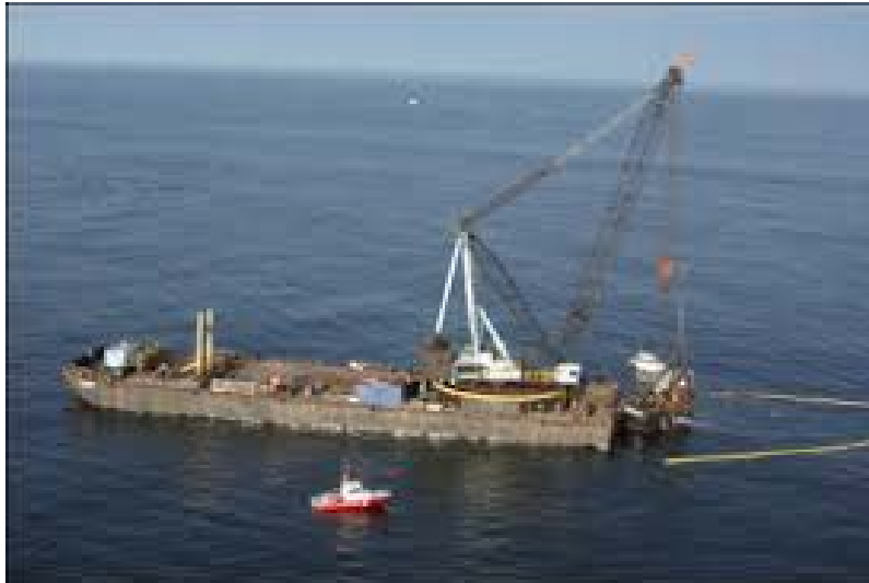
Figure 2-3: Marine Derrick (Barge Mounted Crane)
