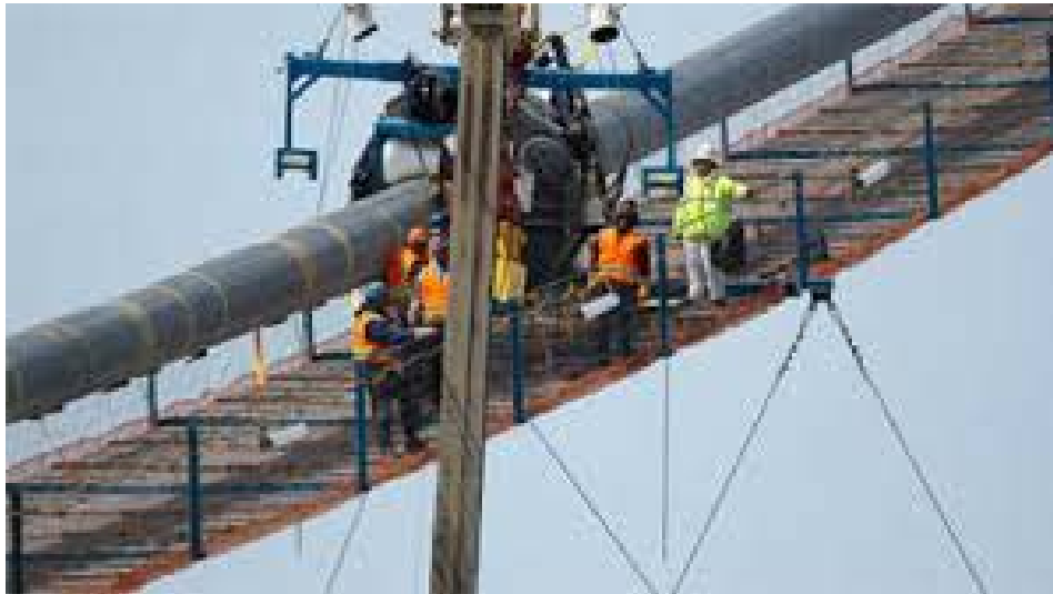
Figure 2-9: Final Cable Wrapping
