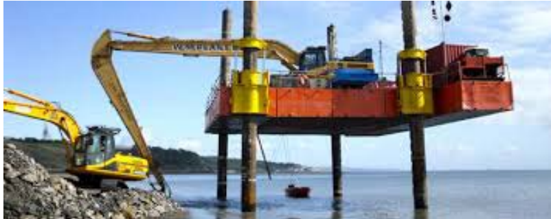
Figure 4-2: Typical Jack-Up barge ( www.cmp.uk.com )
