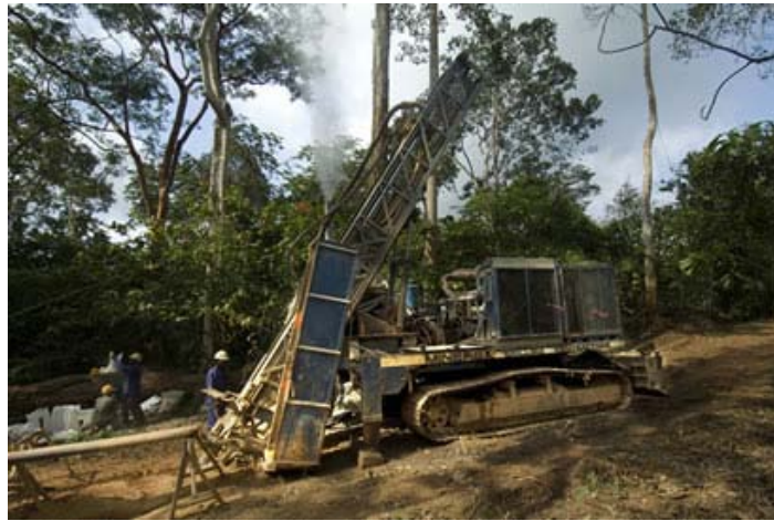
Figure 6-2: Typical Drilling Rig on Tracks
