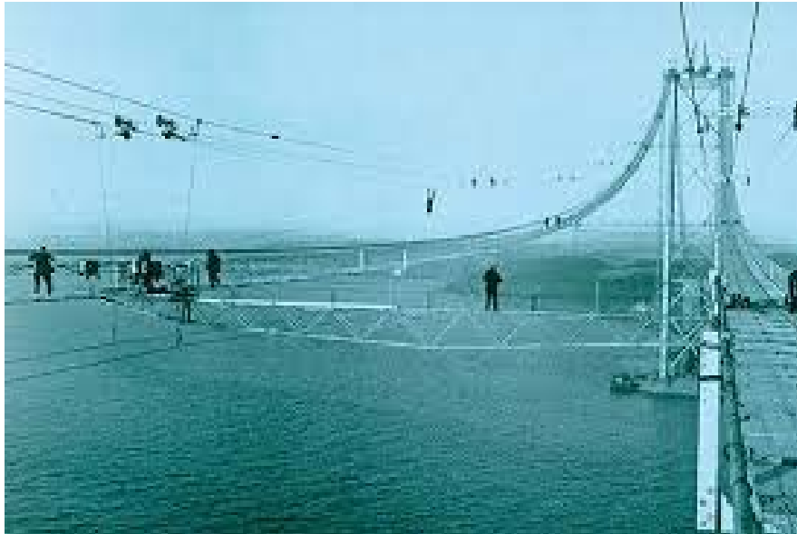
Figure 2-7: Spinning of Main Suspension Cable
