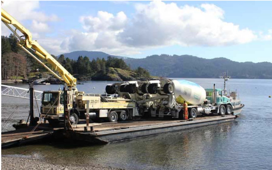
Figure 2-5: Barge Loaded with Concrete Pump Truck and Concrete Trucks
