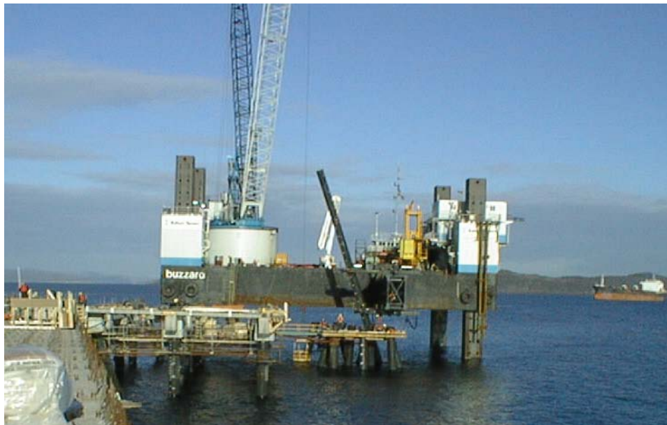
Figure 2-1: Elevated Jack-up Barge in Operation
