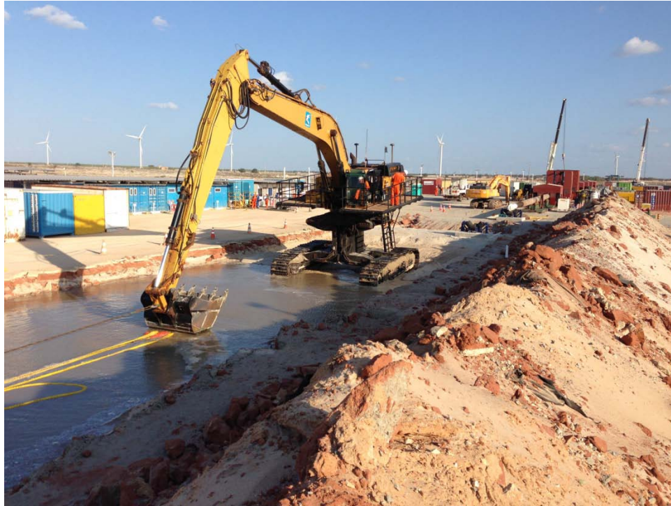
Figure 4-6: Typical Elevated Backhoe (www.jandenul.com)
