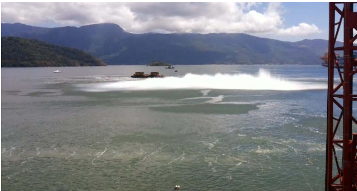
Figure 4-11: Blasting Operation from the YD007 Vessel (Photo taken October 28, 2014)
