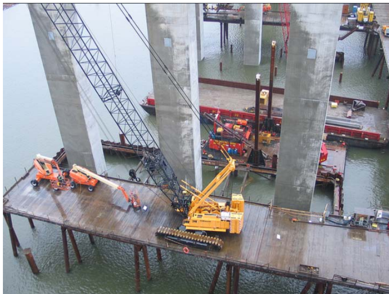
Figure 2-2: Temporary Pile Supported Work Platform
