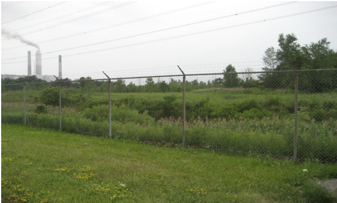
Figure 3.1.4 W - West Site (looking north from Oil Springs Line – July 2012)
