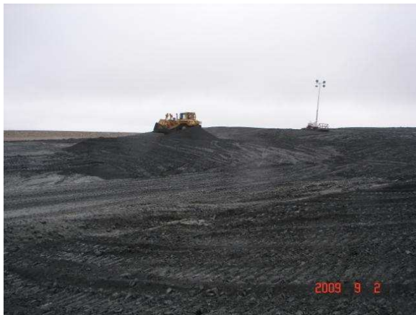
Photo 2-2 Deposition of Dewatered Tailings at Raglan Mine, Xstrata Nickel
