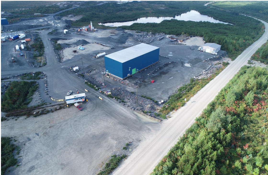
Figure 2. Mining Equipment Garage – Whabouchi Site, September 2024
