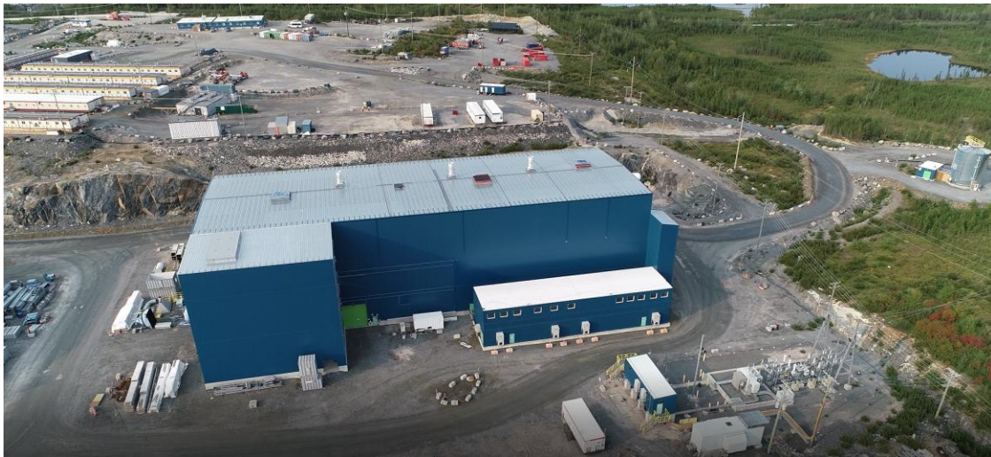
Figure 10. Road Loop Leading to the Concentrator (Eastern Portion) –Whabouchi Site, September 2024
