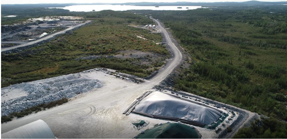
Figure 4. Mining Road Leading to the Explosives Magazine –Whabouchi Site, September 2024
