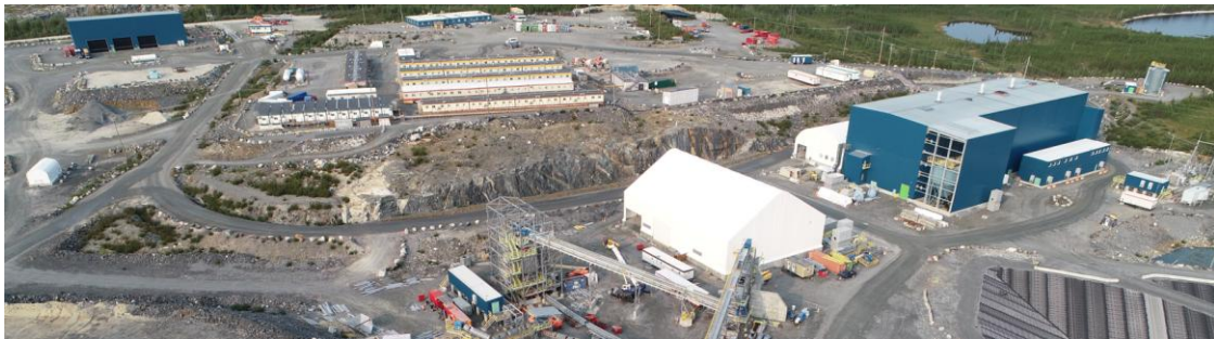
Figure 9. Road Loop Leading to the Concentrator (Western Portion) –Whabouchi Site, September 2024
