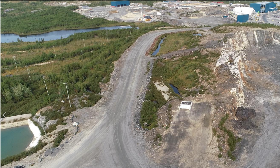
Figure 6. Mining Road Leading from the Pit to the Viaduct – Whabouchi Site, September 2024
