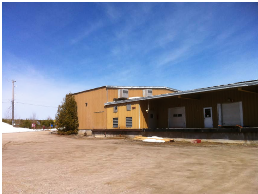
Figure 1.3 Goliath Gold Project Office (Main Warehouse)
