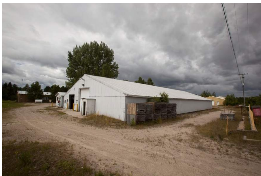
Figure 1.6 Goliath Gold Project Warehousing Infrastructure
