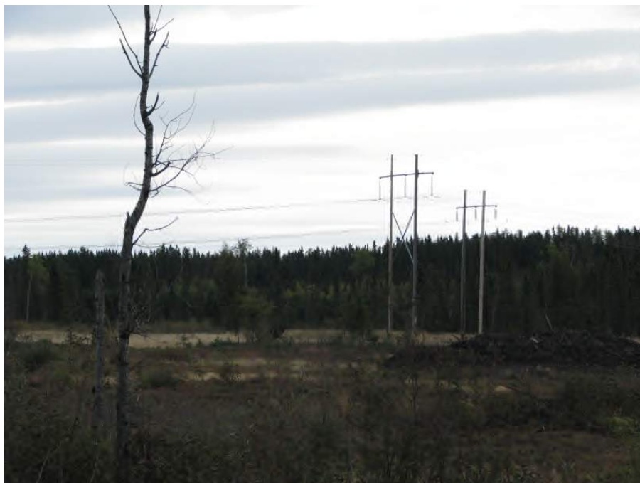
Figure 2.11 Power Line Infrastructure
