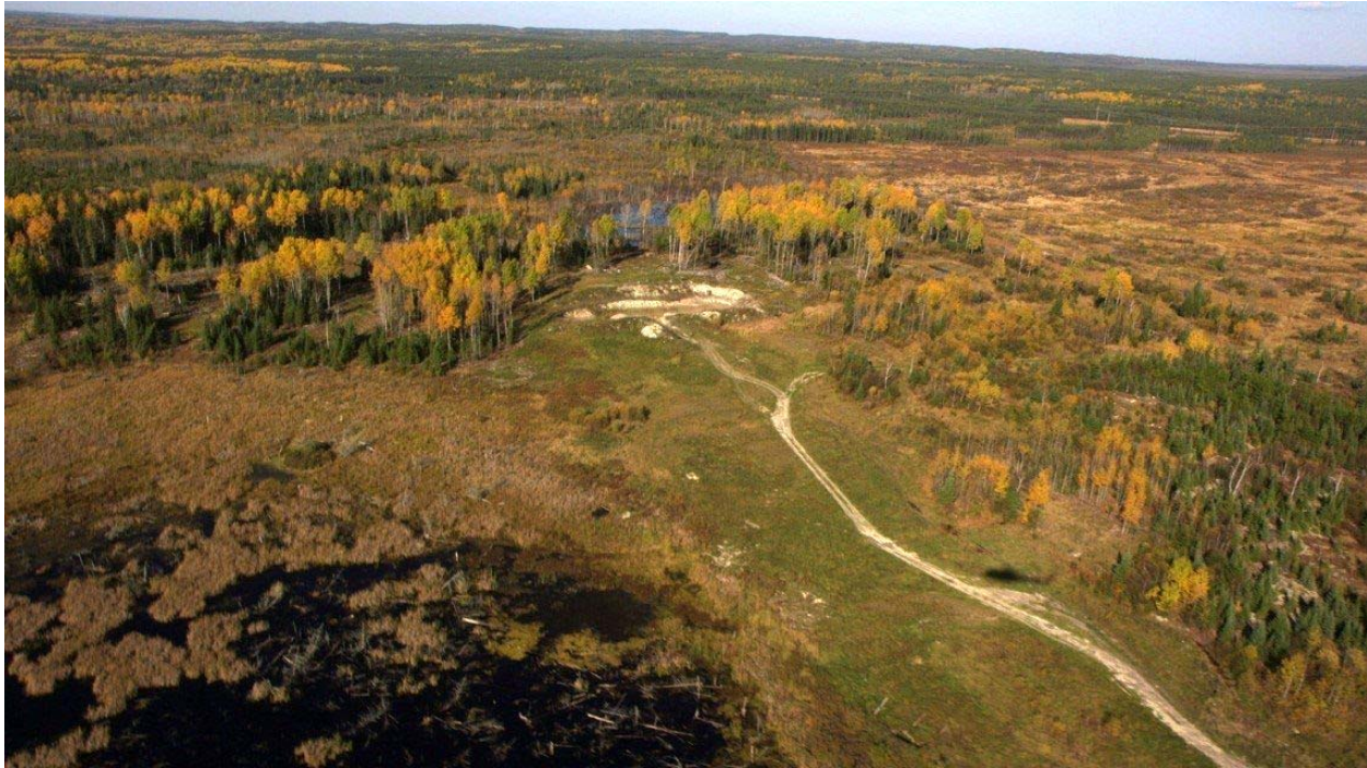
Figure 3.3.1-1: Aerial View of Proposed Open Pit
