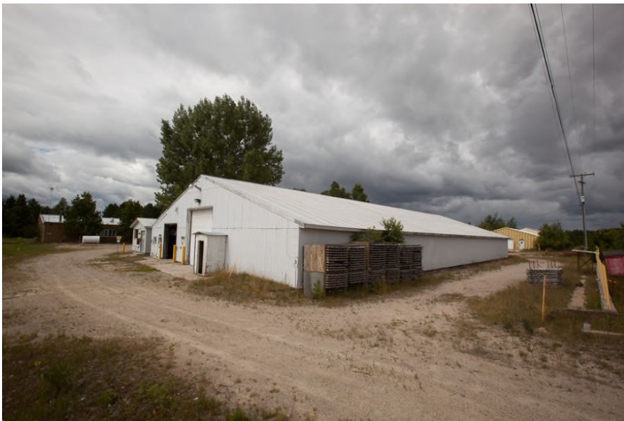
Figure 1.6 Goliath Gold Project Warehousing Infrastructure
