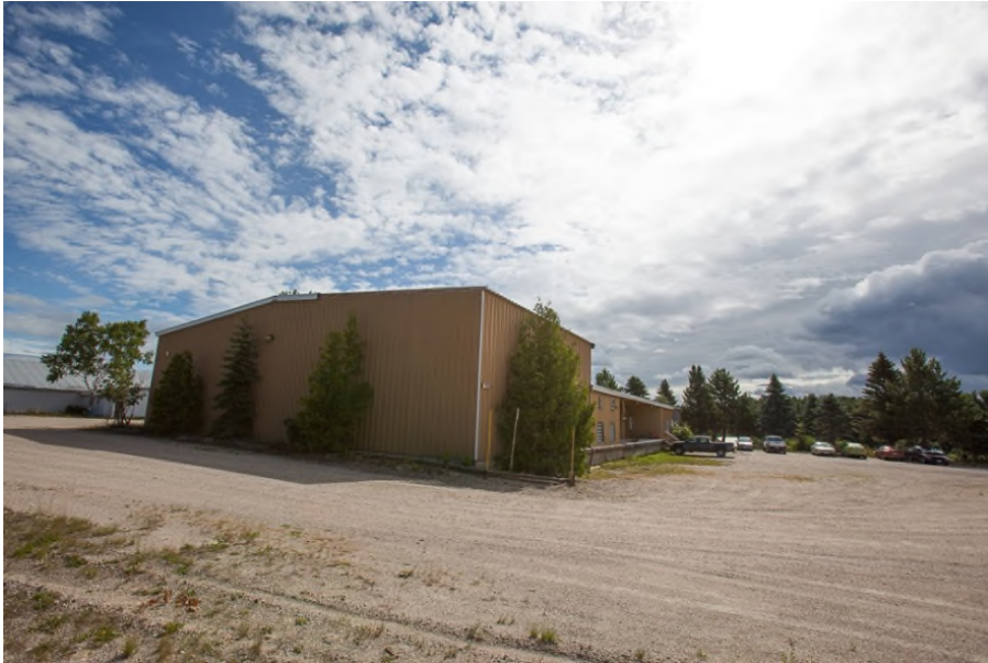
Figure 1.5 Goliath Gold Project Office (Main Warehouse)
