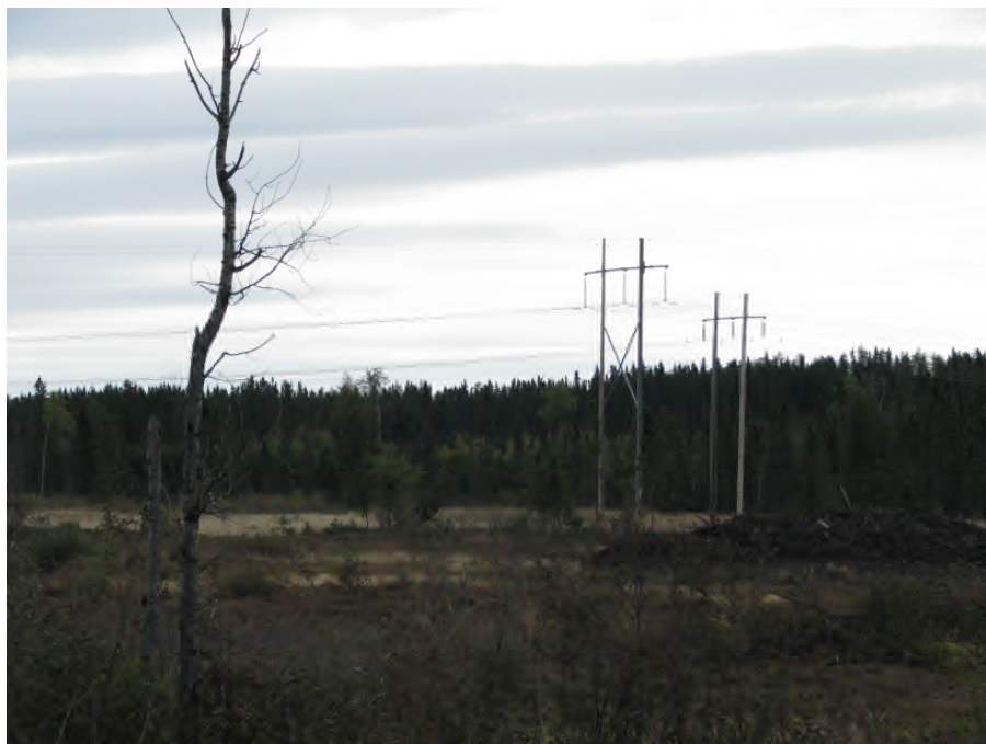
Figure 2.11 Power Line Infrastructure
