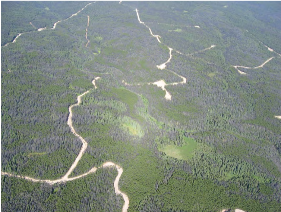
PHOTO 4 – Site of Proposed Site C Main Dam (View to the northwest)
