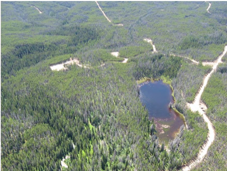
PHOTO 3 Proposed North Abutment of Site D Main Tailings Dam (view to the south)
