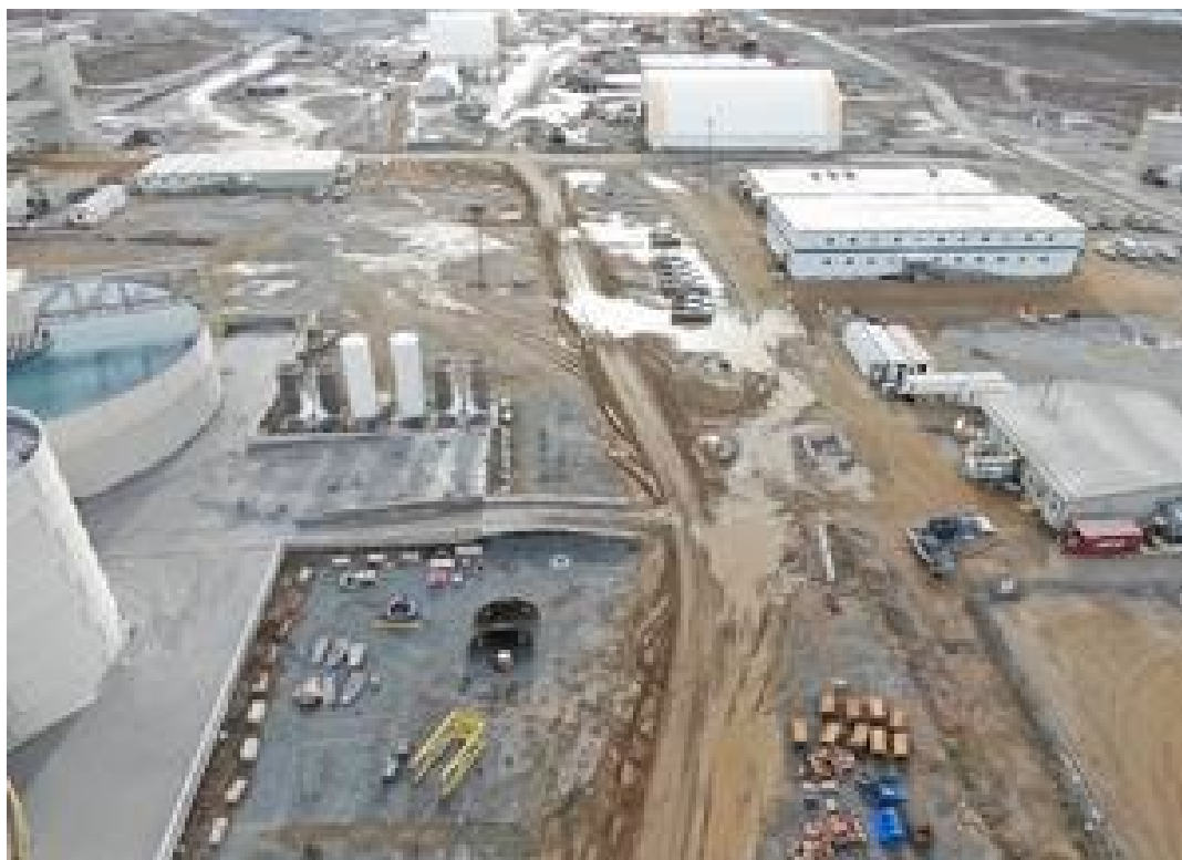
Figure 4. Rainy River Mine Aerial view, looking South-west, 2023
