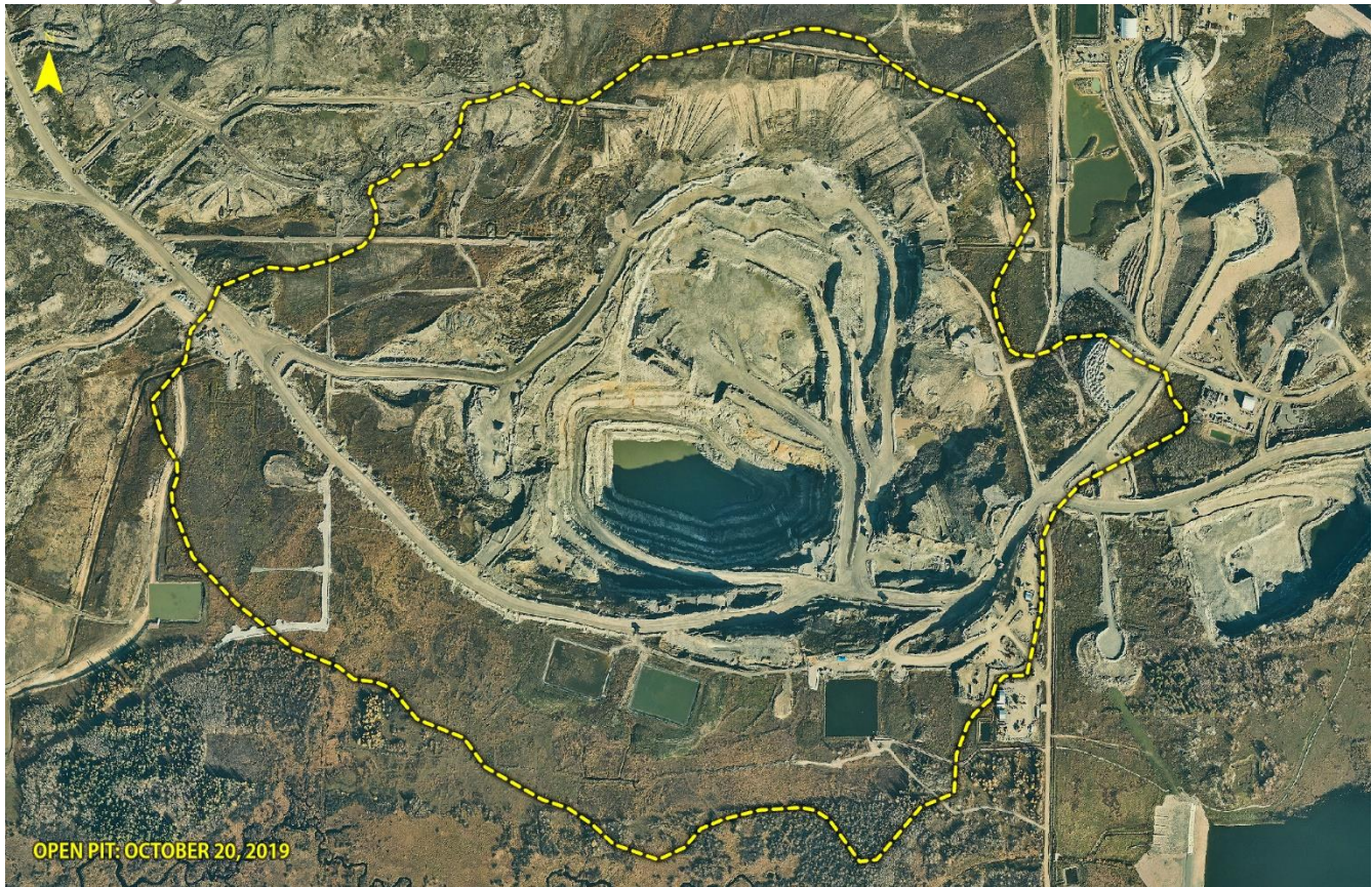
Figure 7: Open Pit Mine aerial imagery October 2019 with final pit shell in yellow
