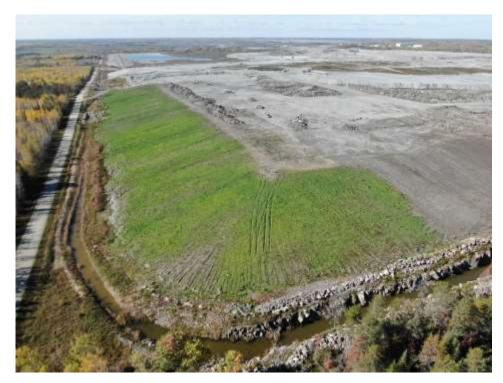
Figure 20. Hydroseed progression on the Southeast EMRS slope (Oct 12, 2021).
