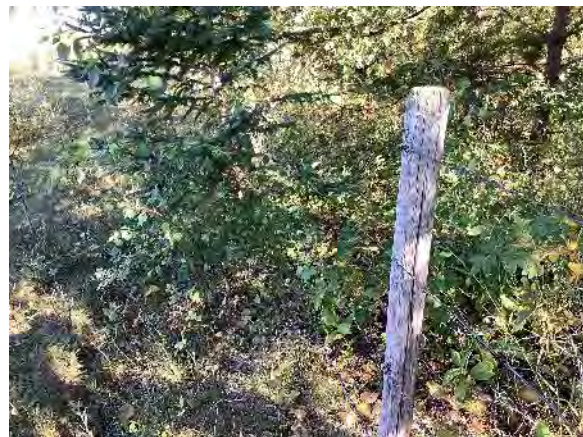
Photo 18: Fence at south boundary of Field 1 in poor condition
