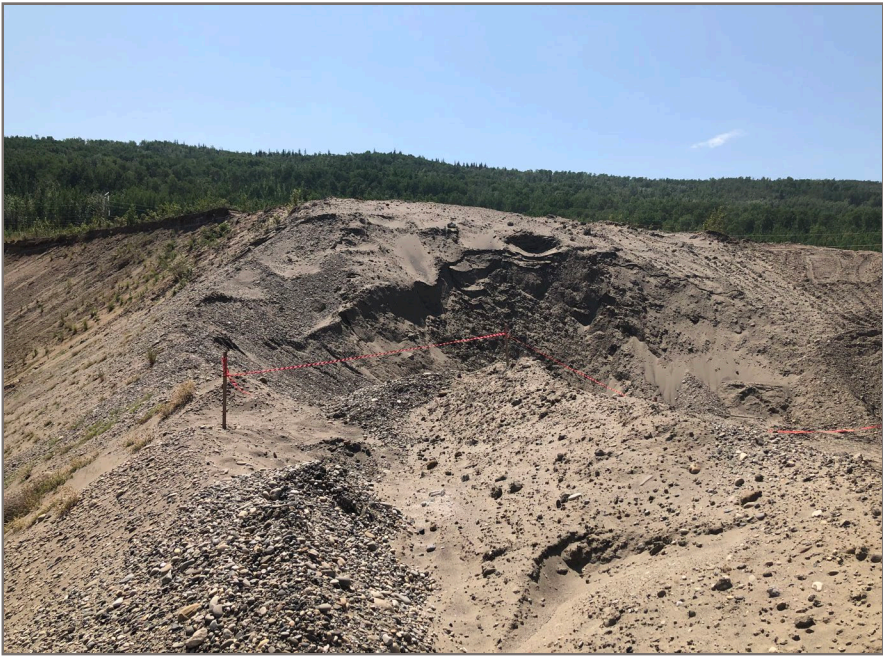
Photo 1: View of the disturbed north-facing slope at the Batch Plant.
