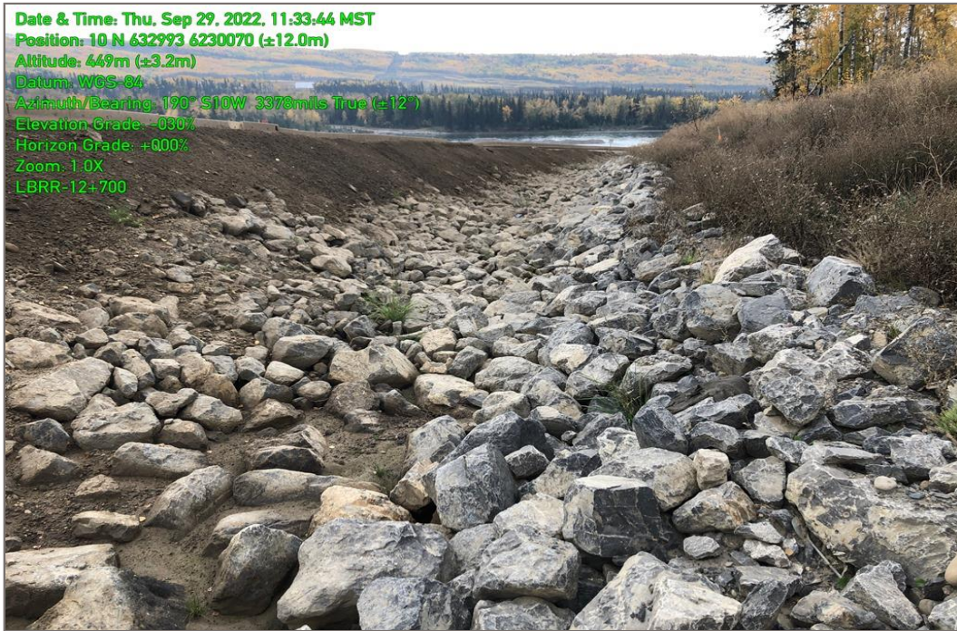
Photo 5: River Road LBRR-12+700 location, September 2022.
