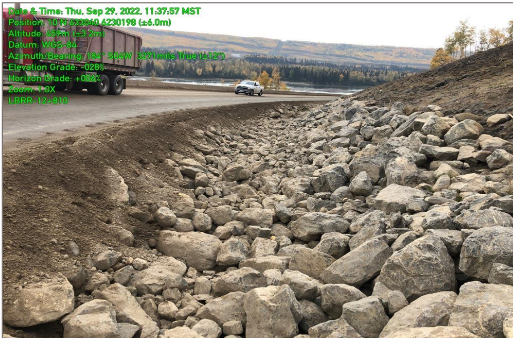
Photo 4: River Road LBRR-12+810 location, September 2022.
