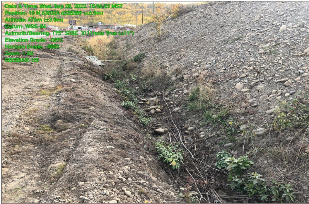
Photo 13: RBSBIAR-US location, looking upstream, September 2022.
