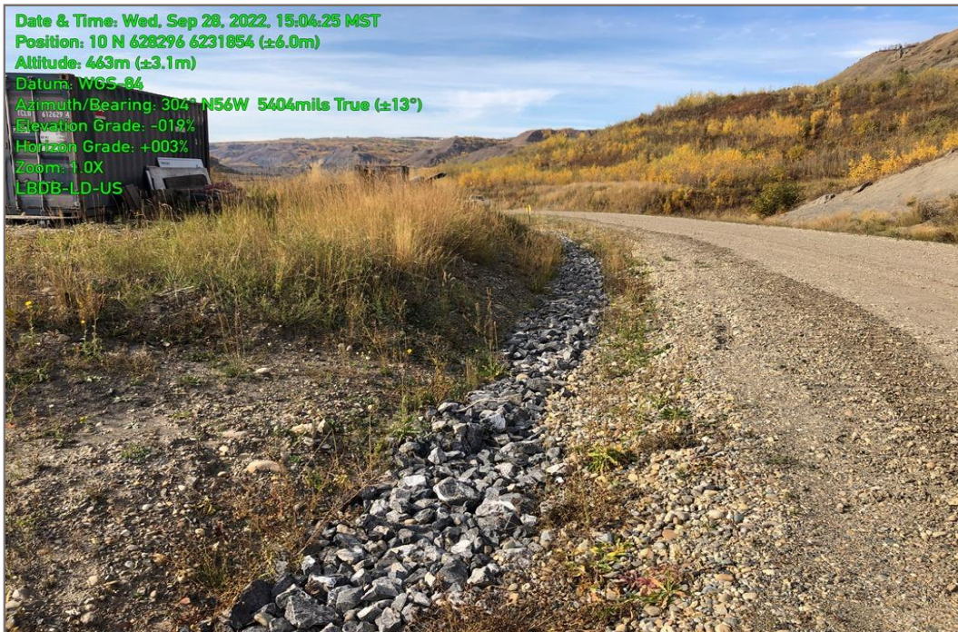
Photo 28: LBDDB-LD-US location, September 2022.
