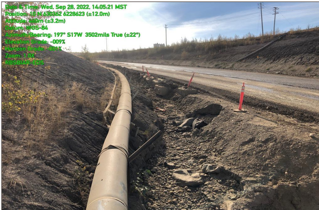
Photo 20: RBSBIAR-EDS location, looking upstream, September 2022.
