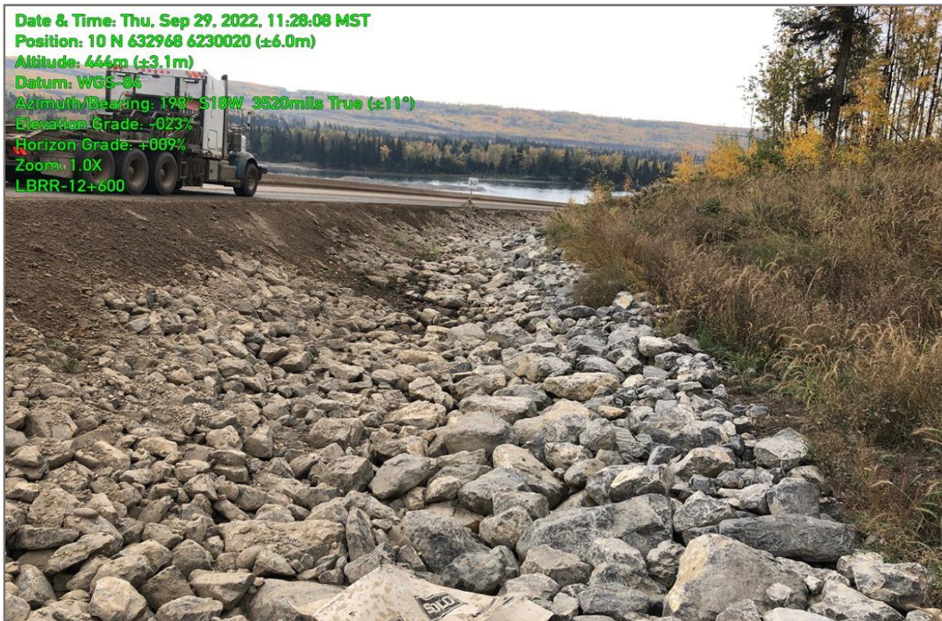
Photo 6: River Road LBRR-12+600 location, September 2022.
