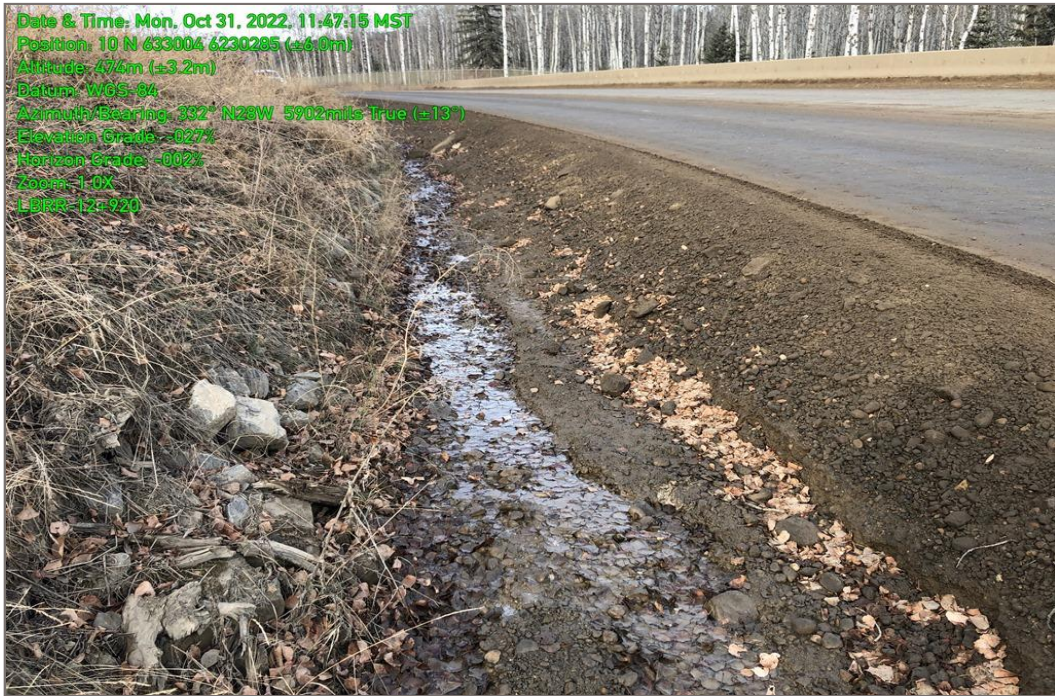
Photo 3: River Road LBRR-12+920 location, October 31, 2022.
