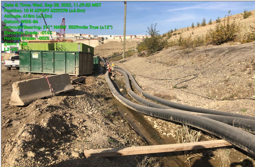
Photo 21: L2-US location, looking northwest, September 2022.
