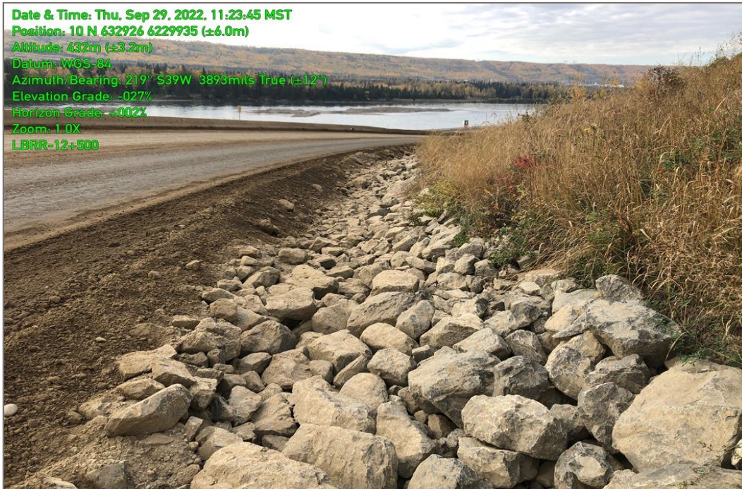
Photo 7: River Road LBRR-12+500 location, September 2022.
