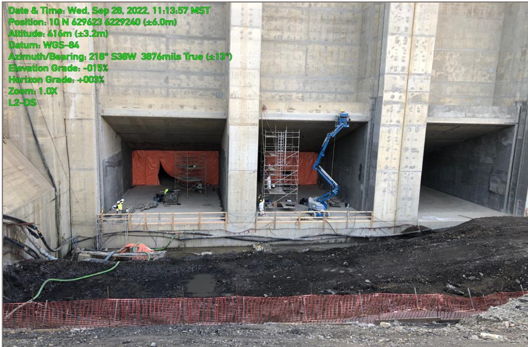
Photo 23: L2-DS location, September 2022. Sample collected in corner adjacent to powerhouse walls
