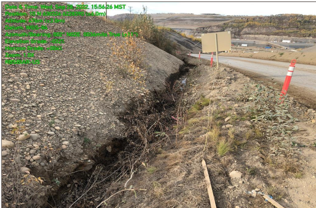
Photo 14: RBSBIAR-US location, looking downstream, September 2022.
