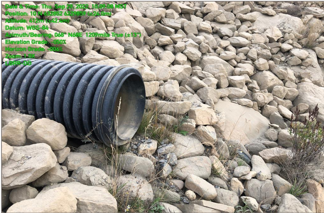
Photo 9: River Road LBRR-DD location, outlet of culvert, September 2022.
