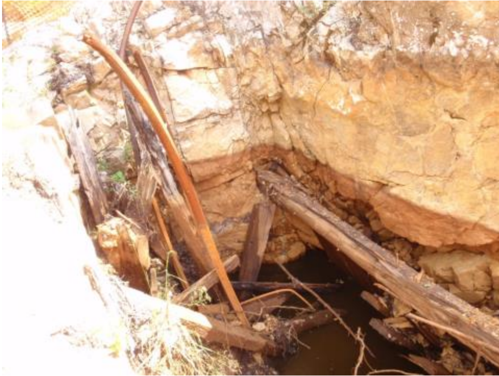
Figure 13: Main Shaft of Sawbill Mine (View North)
