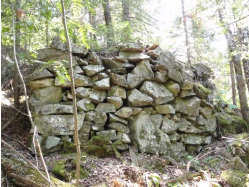
Figure 24: Tramway Abutment for Crossing of a Creek (View Southeast)
