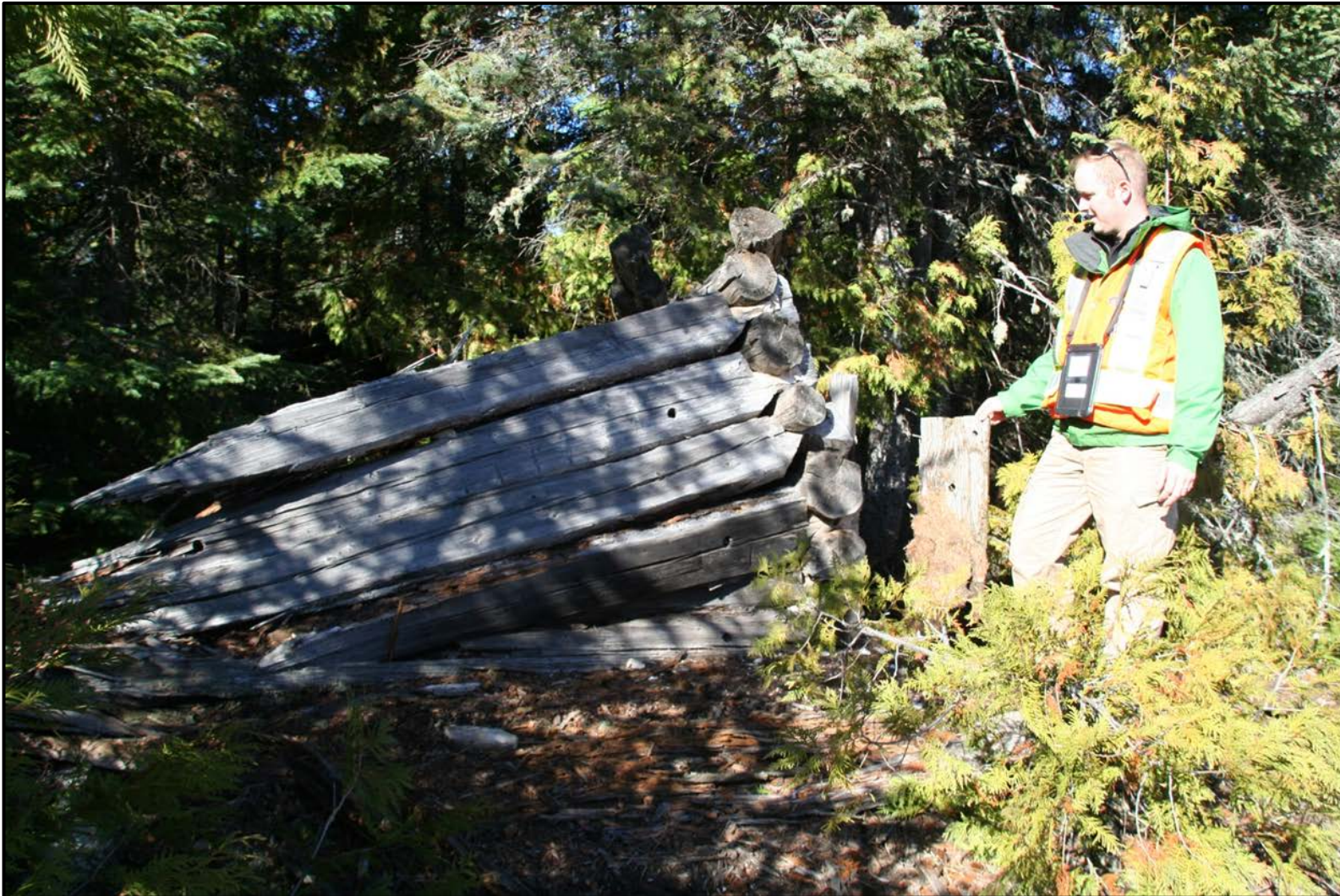
Plate H-8: Mine cabin, corner joints
