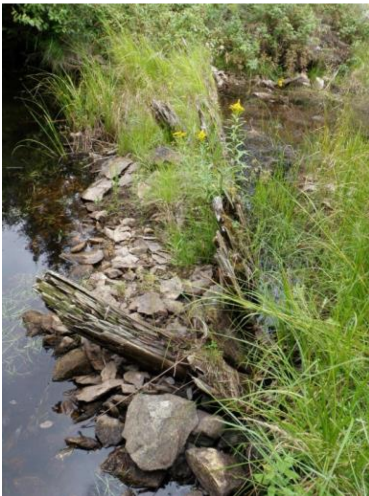
Figure 32: Close up of Timber Crib Dam Structure (View North)
