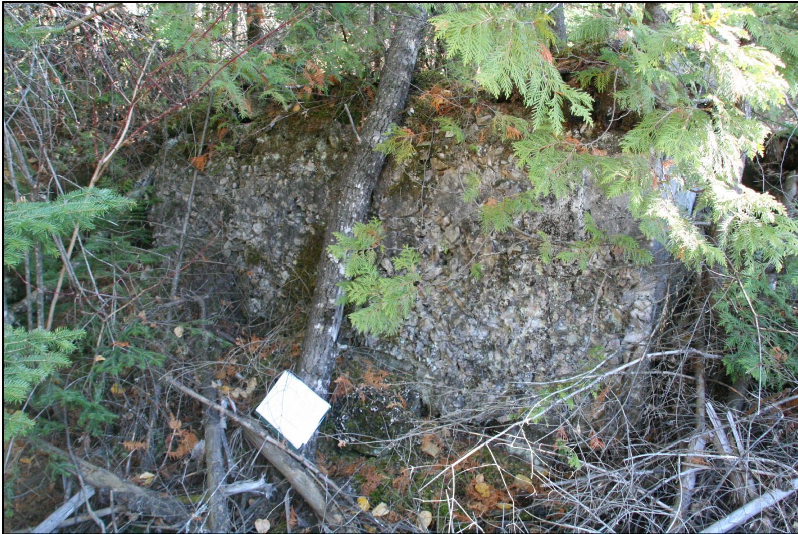
Plate H-14: Concrete machinery base with notebook for scale
