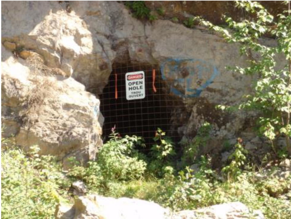
Figure 29: Adit for the Original Hammond Reef Mine (View North)
