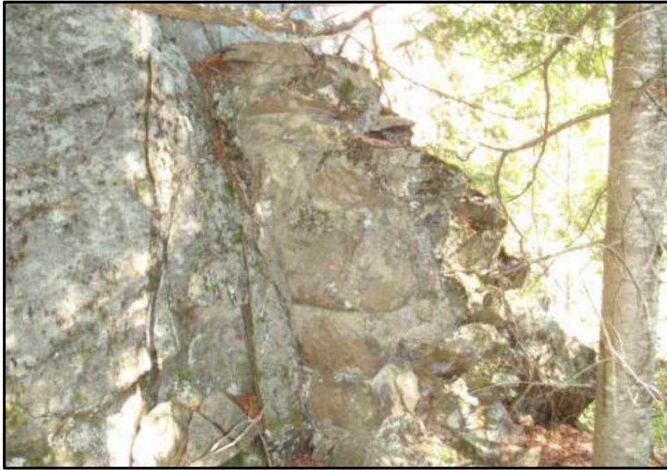
Figure 2: Stone dam remains of former power plant. October 2011. Source Golder Stage 1 Baseline Study and Stage 2 Archaeological Assessment 2013.
