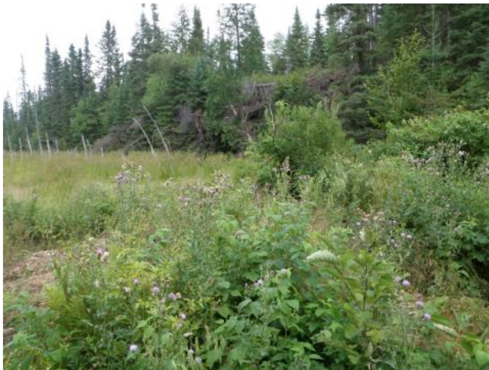
Figure 35: Waste Rock Dam Blocking Main Channel of the Head Pond (View southeast)
