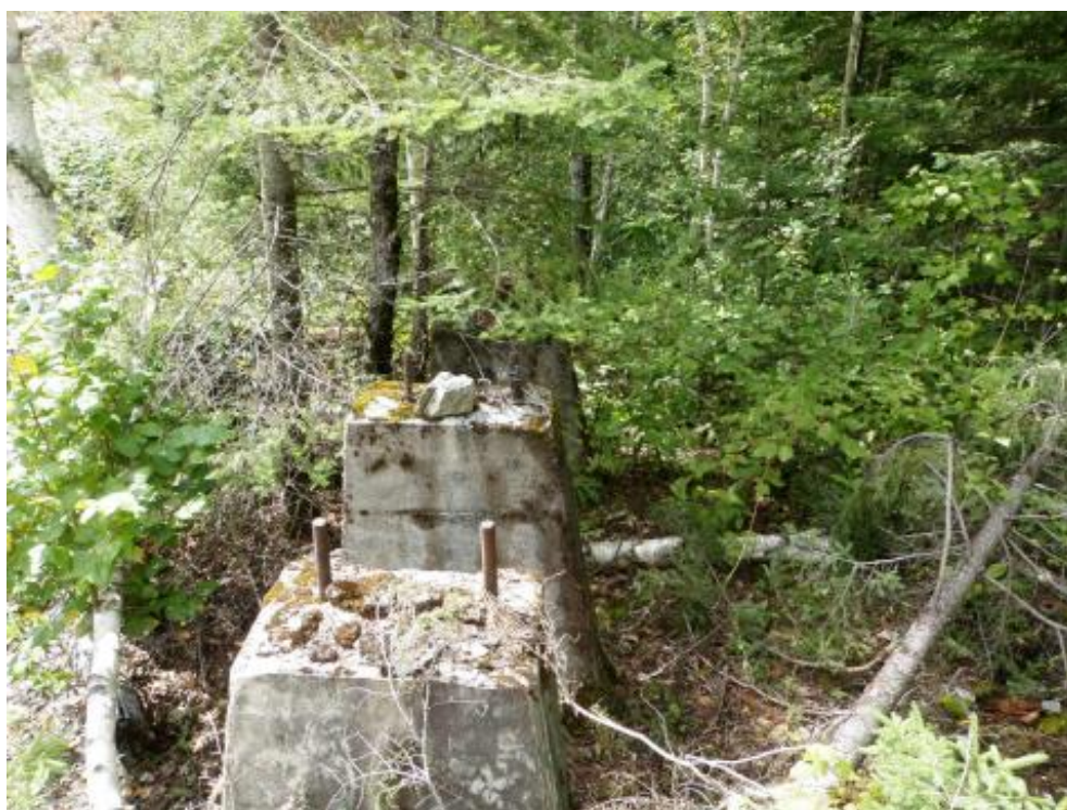
Figure 17: View of Concrete Pedestals in the Central Area of the Stamp Mill (View West)
