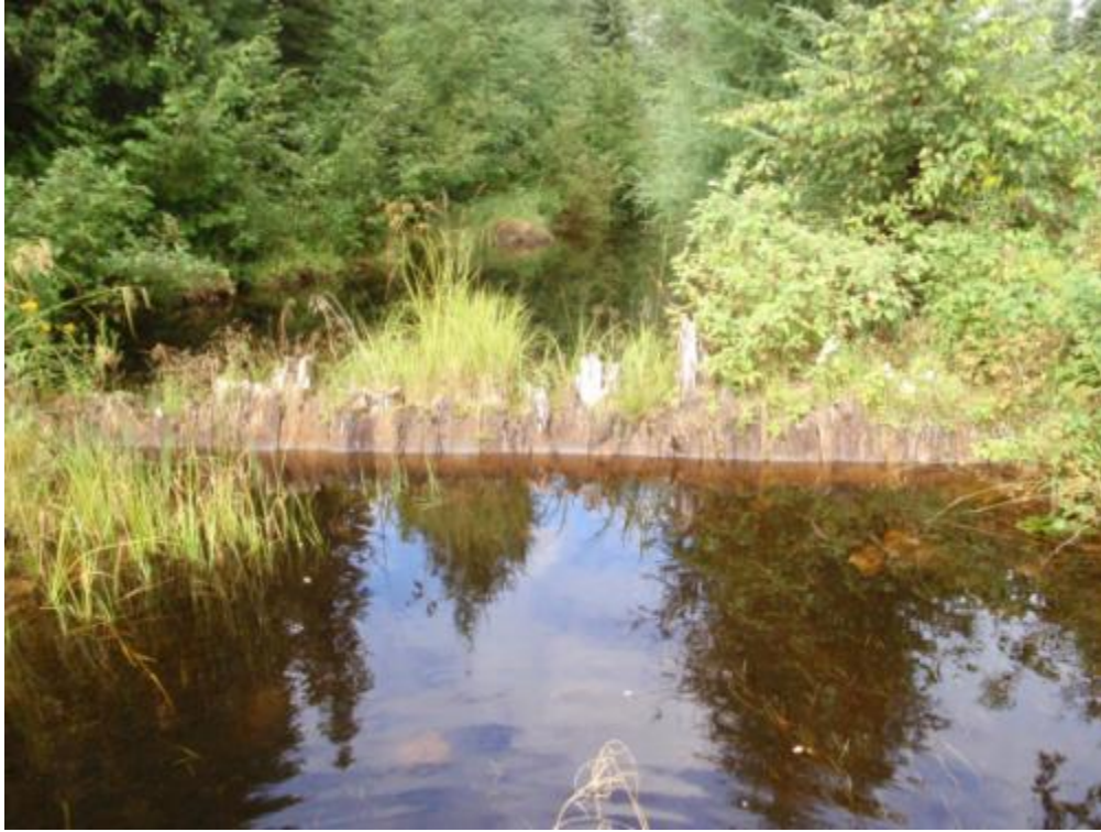
Plate 53: Photo 677, Waypoint k97, Hammond Gold Reef Mine reservoir wood dam, facing southeast
