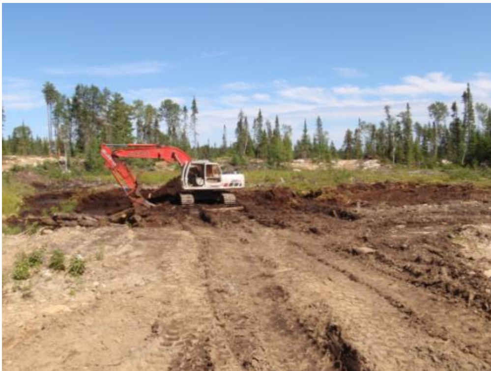
Plate 16: Photo 041, Waypoint P34, backfilling wetlands, facing southeast
