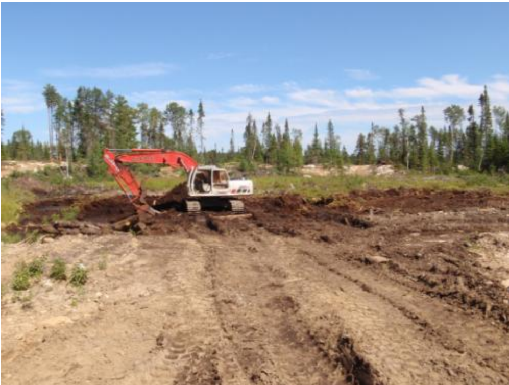
Plate 16: Photo 041, Waypoint P34, backfilling wetlands, facing southeast
