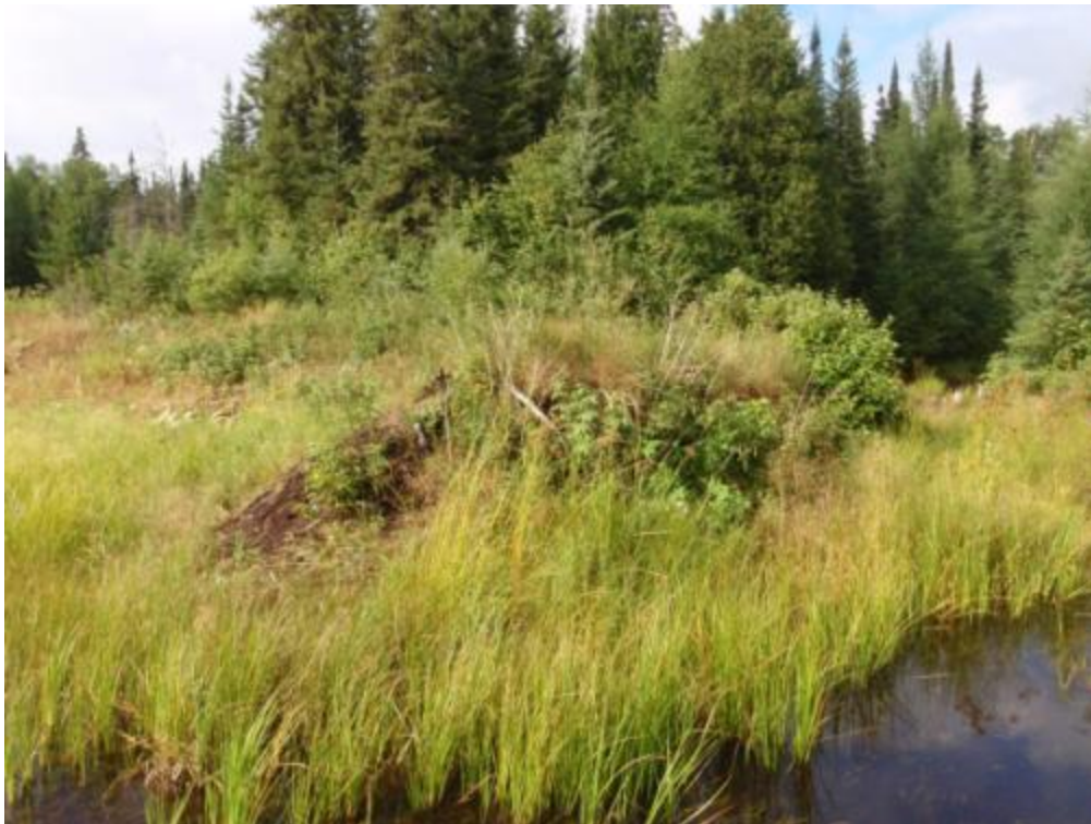
Plate 54: Photo 277, Waypoint k97, Hammond Gold Reef Mine reservoir earth dam, facing east
