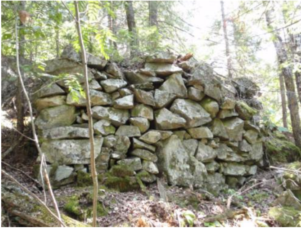
Plate 63: Photo 259, Waypoint R10, field stone footing for tram line, facing east
