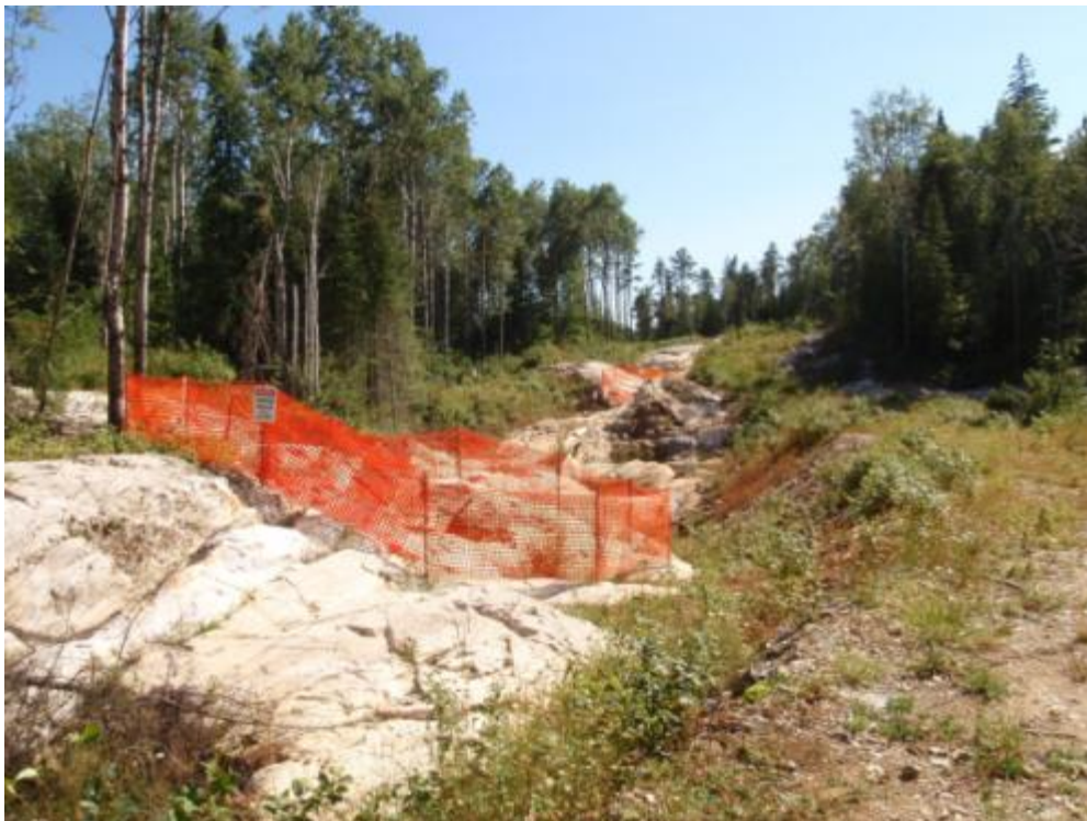
Plate 58: Photo 066, Waypoint 039, mine shafts (in orange fencing), facing northeast
