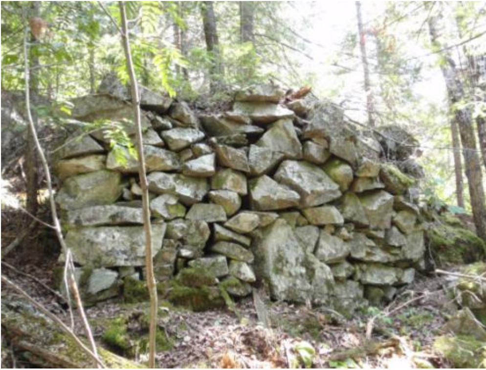
Plate 63: Photo 259, Waypoint R10, field stone footing for tram line, facing east
