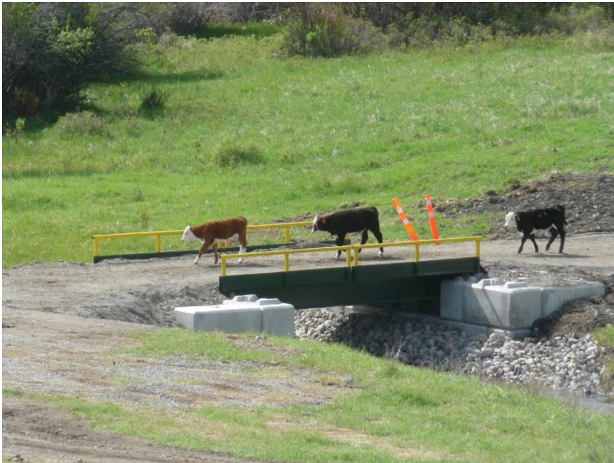
Upgraded Peterson Creek crossing
