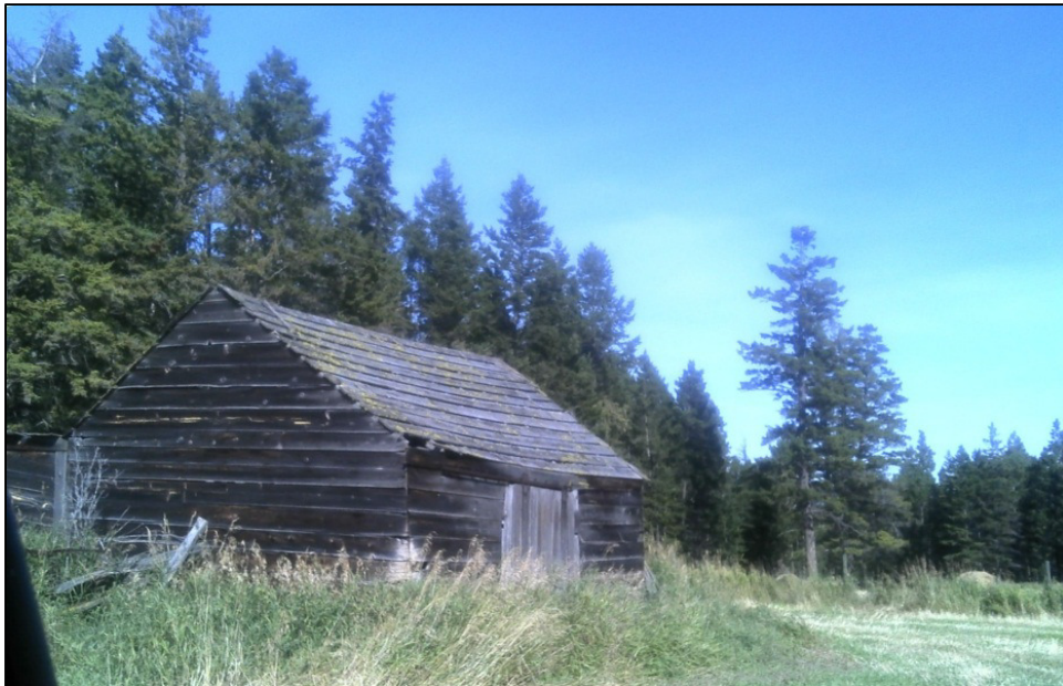
Plate 4.2-4. View of barn and the surrounding area, looking west.
