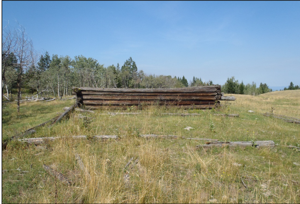
Plate 4.2-12. View west of structure M20-HF2 with extension of logs in foreground.
