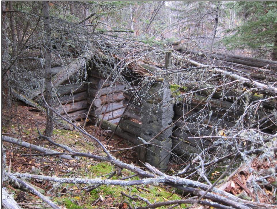
Plate 4.2-8. View of Homestead 2 (AJ14-10-22-H1) looking northwest.
