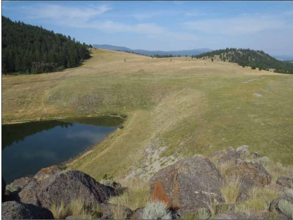
Plate A4-1. View northwest of the proposed Ore Stockpile and the northern edge of the TSF and embankments. Photo taken from ASU Q16.
