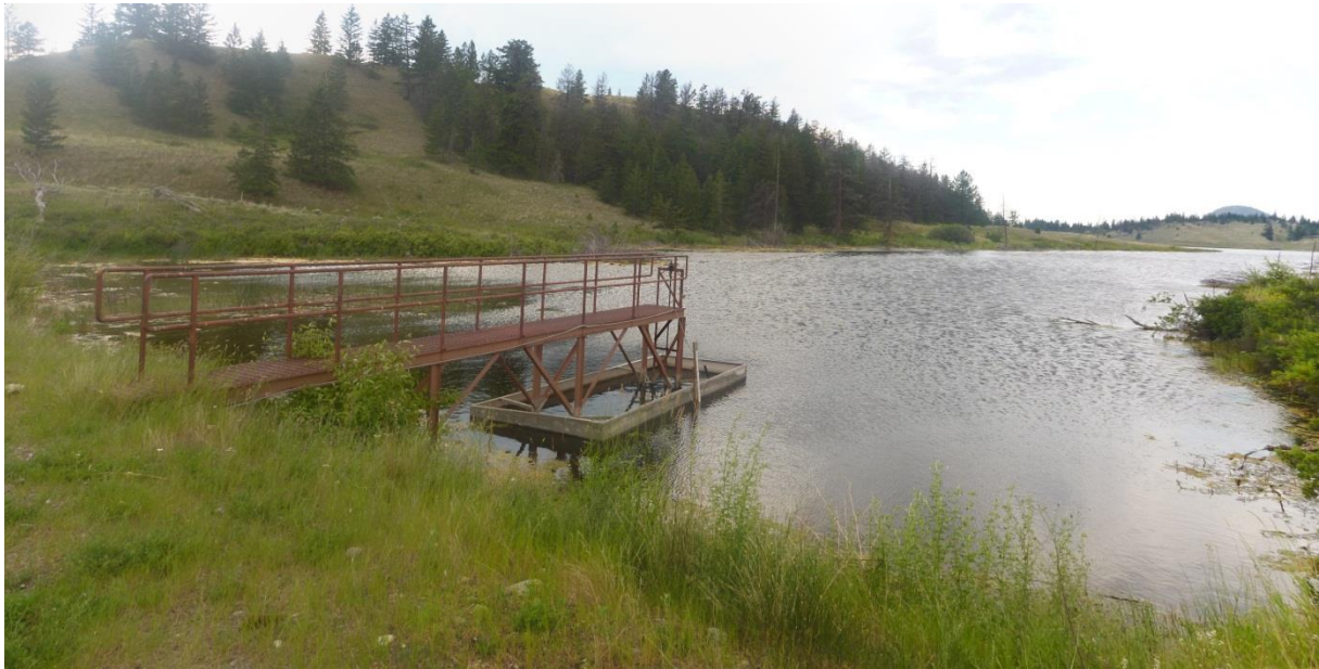
Figure 3-3. Jacko Lake outflow control structure.
