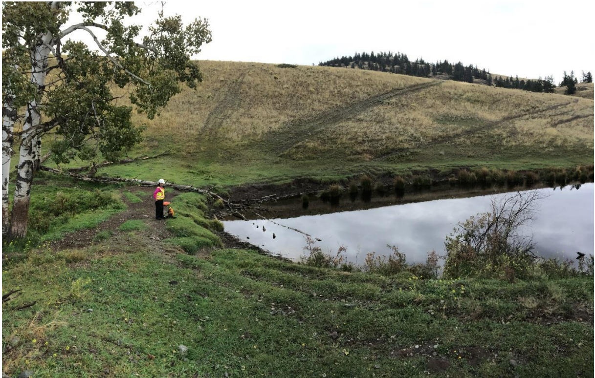
Figure 7-4. Road crossing of Keynes Creek downstream of Goose Lake, which has created a small man-made lake. BGC photograph of September 14, 2014.
