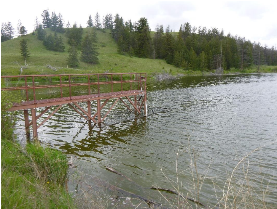
Photo 4. Jacko Lake red platform (spillway overflow control) staff gauge on May 29, 2014. The BGC monitoring station and staff gauge is located in the photo background at the edge of the lake.
