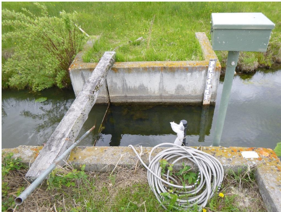
Photo 6. JACSEEP hydrometric station and staff gauge on May 29, 2014.
