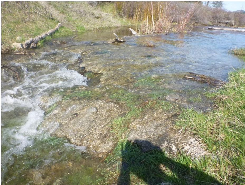
Photo 2. Jacko Lake overflow spillway entrance on May 6, 2014.
