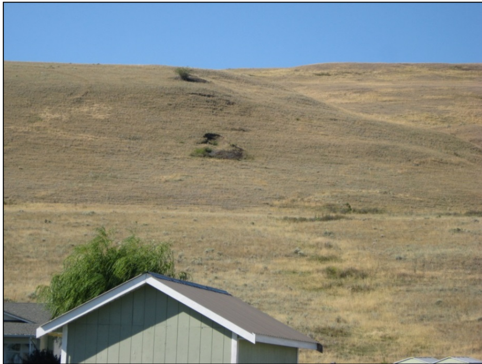
Figure 4.9 Recent Debris Slide in Eolian Sediments (WP 50)
