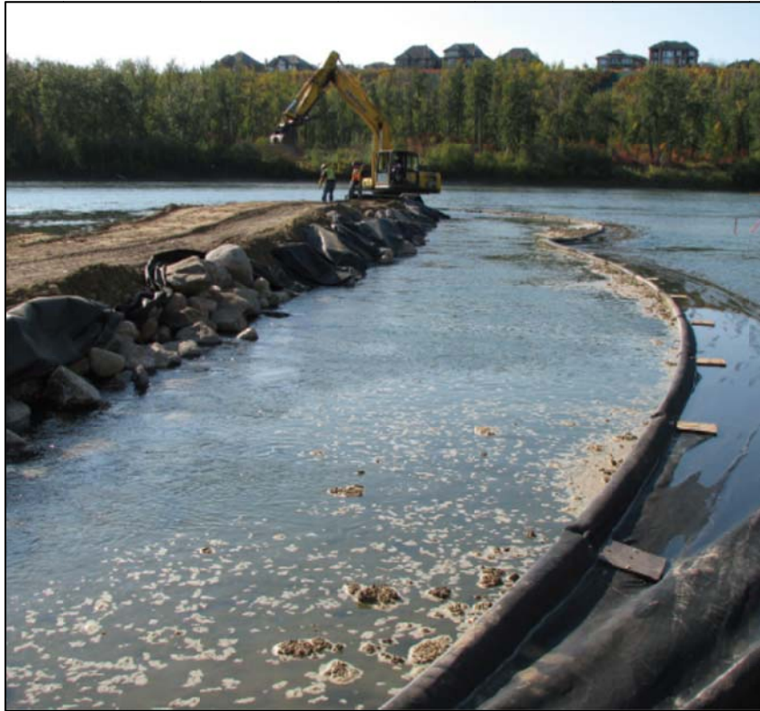
Photo 2 – Floating silt curtain installation (Nilex example)
