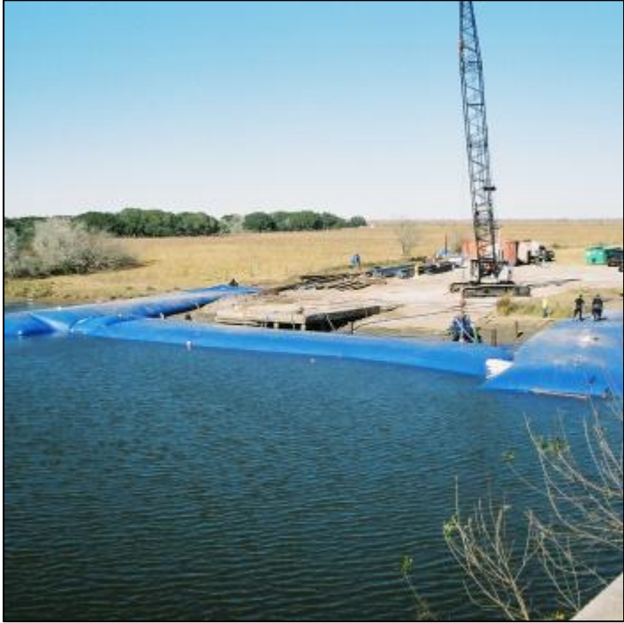
Photo 3 – Temporary water filled dam installation (Nilex example)
