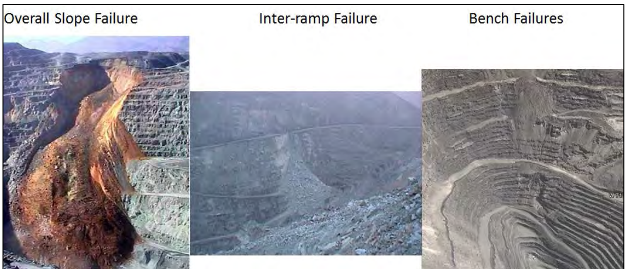
Figure 3-2: Slope failure at different scale
